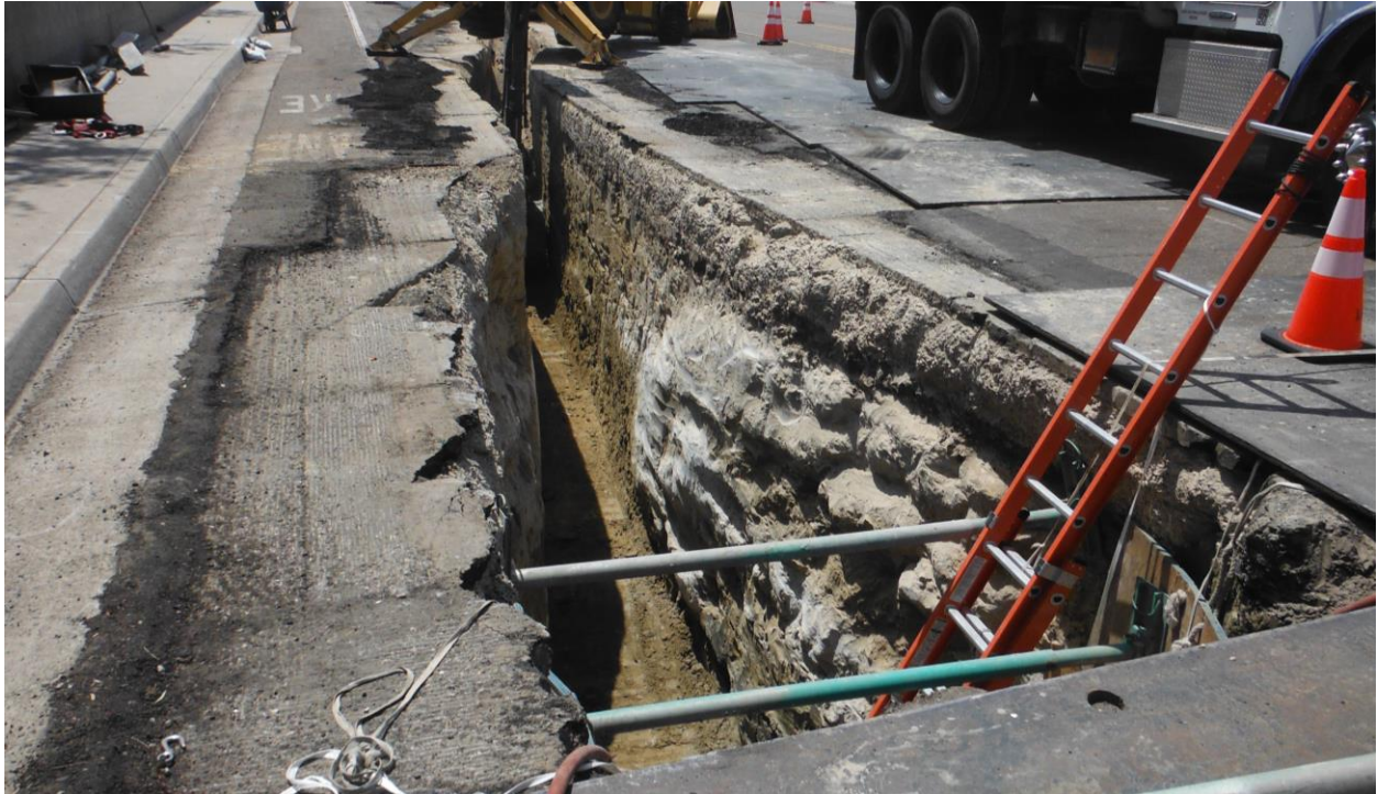
Figure 5. Interfingering deposits of the Friars Formation (light gray) and Scripps Formation (yellowish tan) as exposed during paleontological mitigation of trenching along Murphy Canyon Road. Artificial fill underlying the existing pavement is visible in the uppermost ~1 foot of the trench. Fossilized internal molds of marine mollusks were recently collected in this area from a yellowish gray, fine-grained micaceous sandstone of the Scripps Formation. Photo taken by Bradford O. Riney, 8 May 2018.
