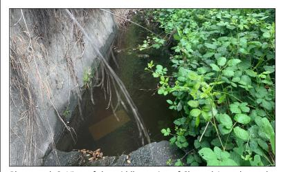
Photograph 3: View of the middle portion of Channel A on the study area, facing northwest (upstream). Note vegetation and sediment to the right and cracked concrete channel bottom to the left.
