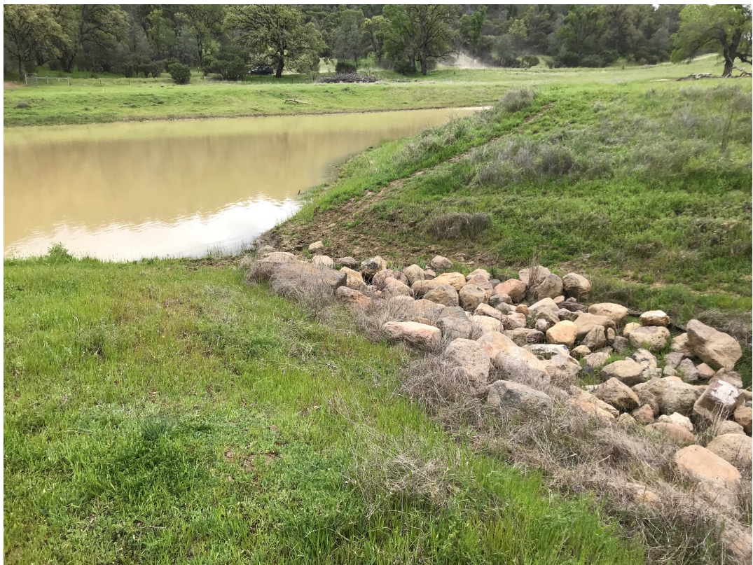
Dam and engineered outfall of stock pond
