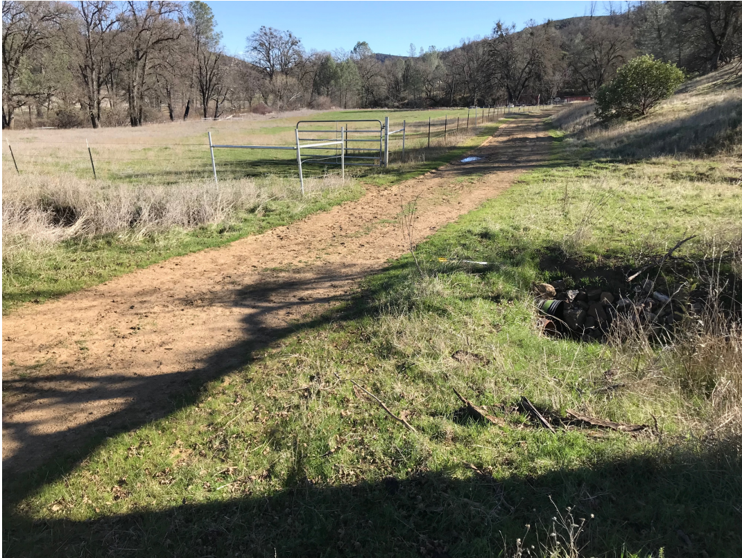
Access road and culverted watercourse crossing between existing and proposed cultivation areas
