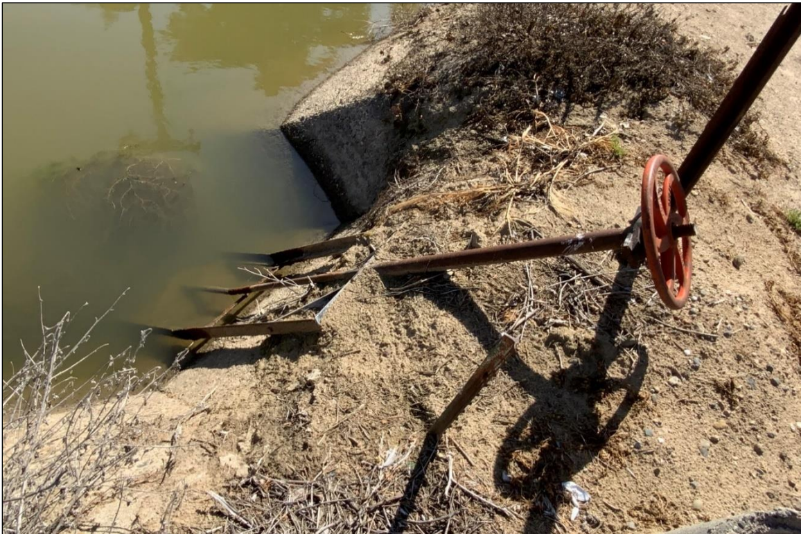
Figure 4-9 Dilapidated water gate feature with deteriorating concrete lining.
