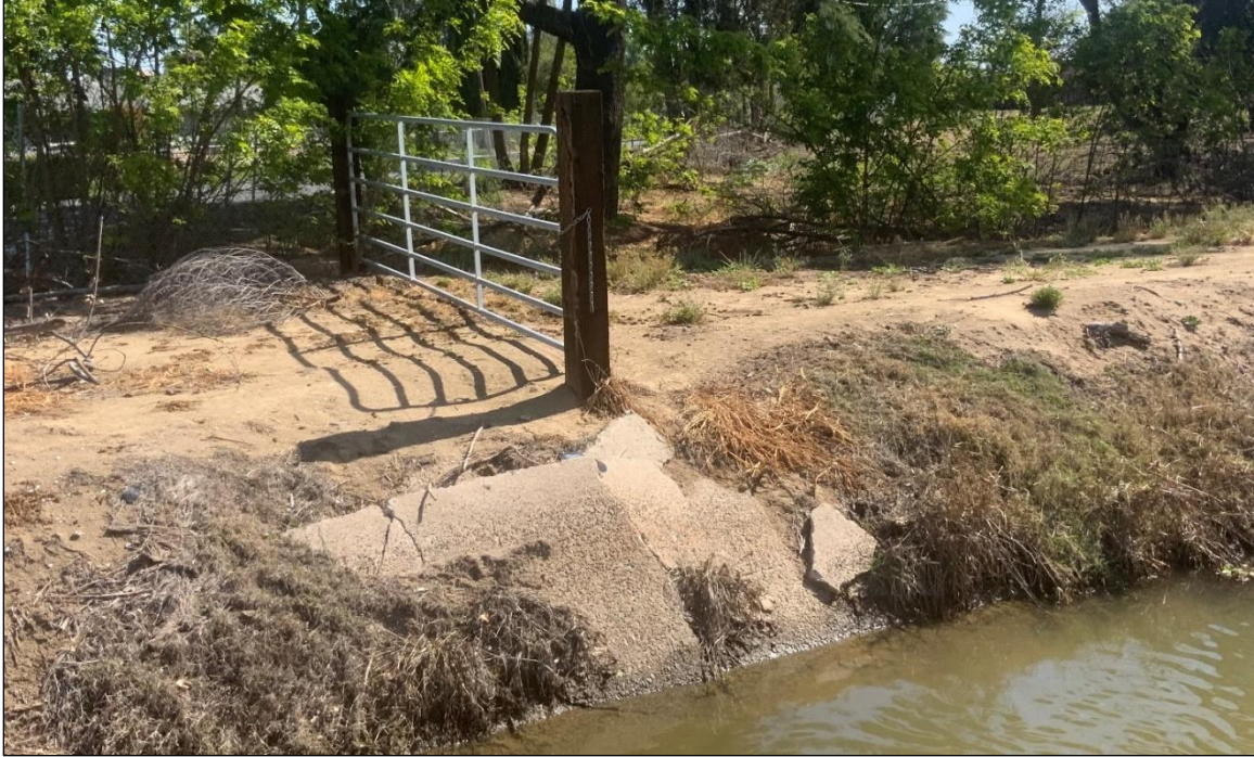
Figure 4-12 View of the farm gate on the east levee with evidence of cracking concrete lining along the bank, facing east.
