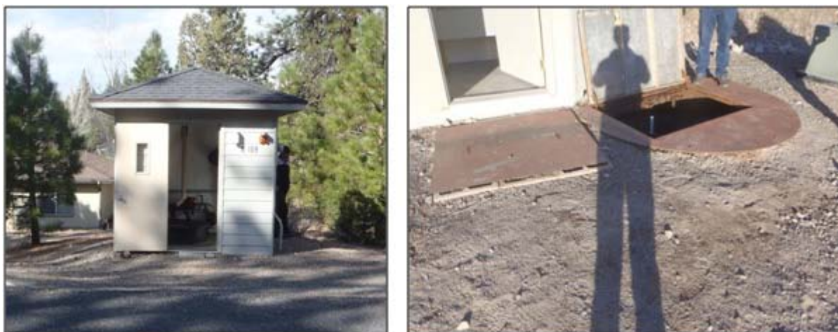
Figure 3-4. Typical steel wet well located inside building, B-109 (left), and outside building, B-114 (right).
