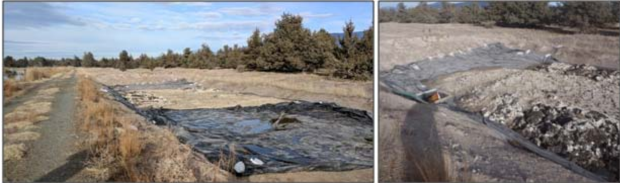
Figure 3-9. Temporary sludge drying bed with trench drain and 100 gallon sump.
