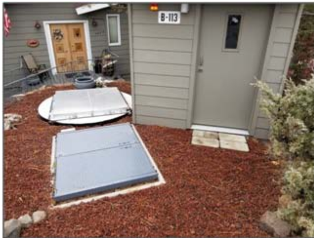
Figure 3-2. Typical concrete wet well and cover (B-113).
