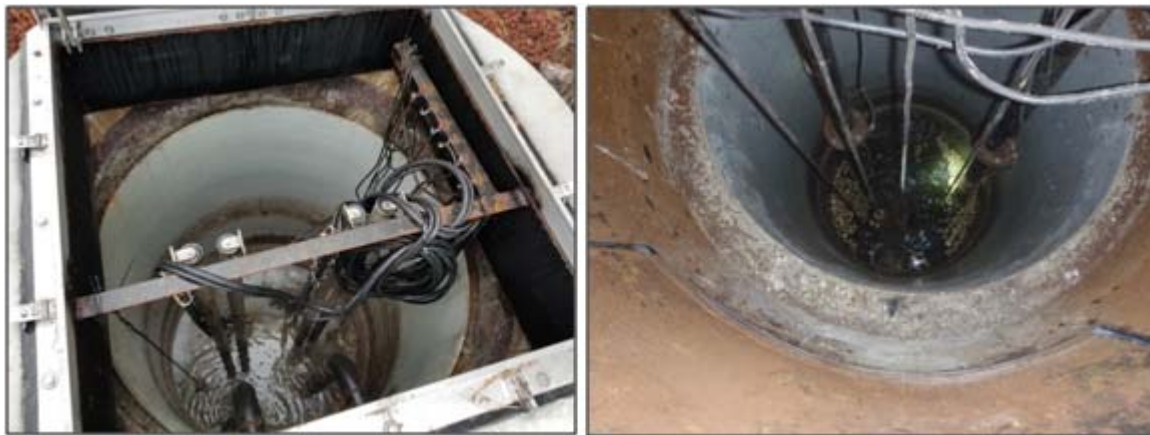
Figure 5-3. Rehabilitated concrete wet well, B-113 (left), and steel wet well, B-103 (right).
