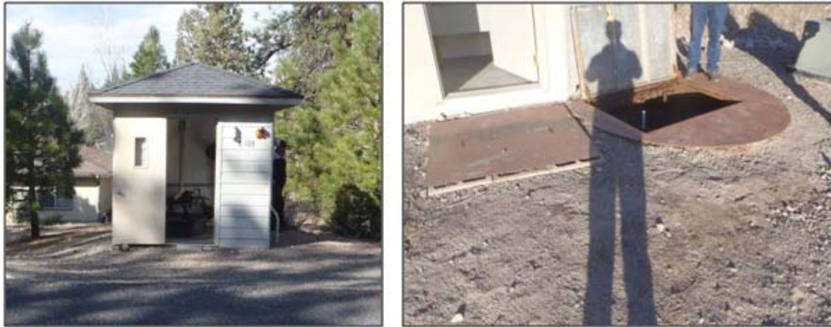
Figure 3-4. Typical steel wet well located inside building, B-109 (left), and outside building, B-114 (right).
