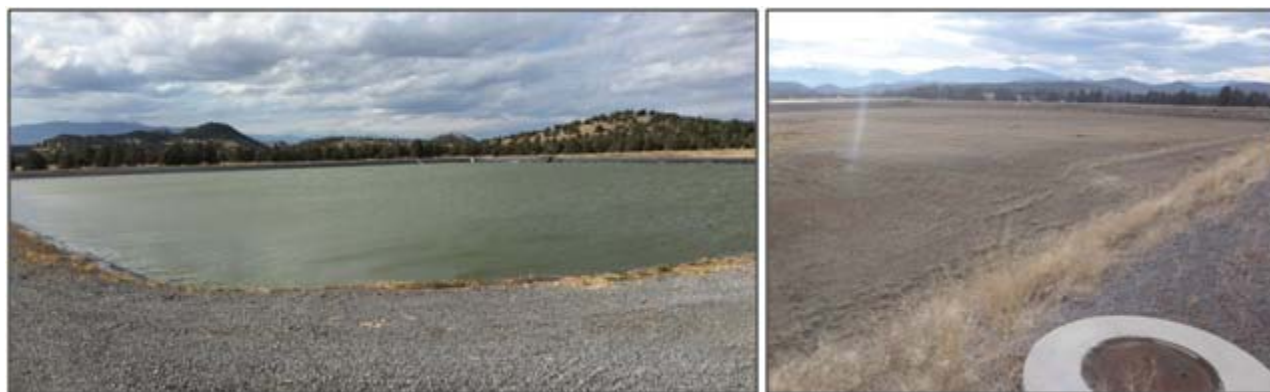
Figure 3-8. Pond 4 (left) is currently lined, whereas Pond 5 (right) is to be lined.
