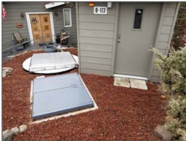
Figure 3-2. Typical concrete wet well and cover (B-113).
