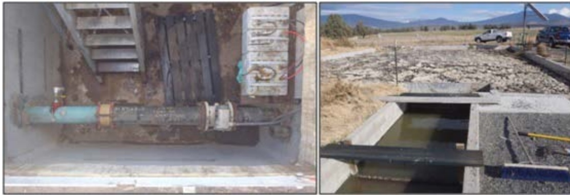
Figure 3-5. Flow meter vault (left) and primary tank (right) at WWTF.
