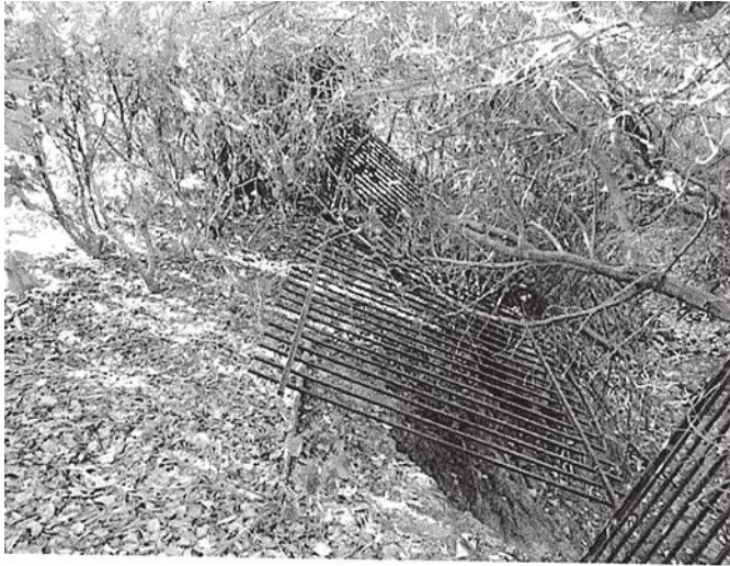
Photo 9 (Courtesy of W. McGuire): Upstream view of the eroded west bank through a failed section of the existing
