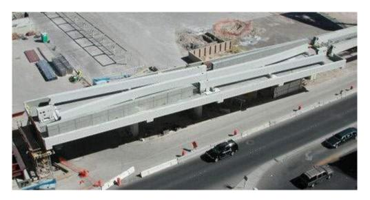
Figure 7-8: Monorail X-Crossover Example, Las Vegas Monorail System (Image Source: LRN Library)
