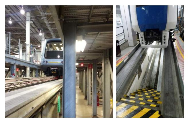
Figure 8-3: Example Light Maintenance Access
