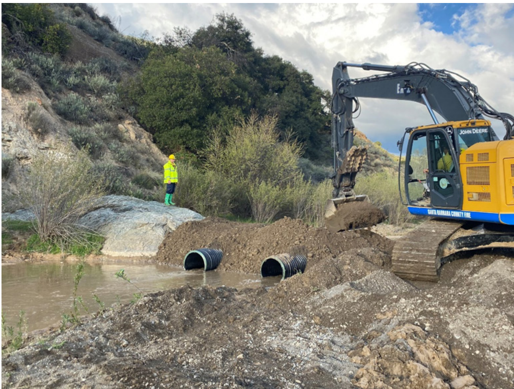
Installed berm and underflow pipes to control spilled oil from traveling downstream
