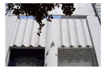
Figure 8. Molded chevron-profile stucco pattern above openings at the 63 Brady Street volume.
