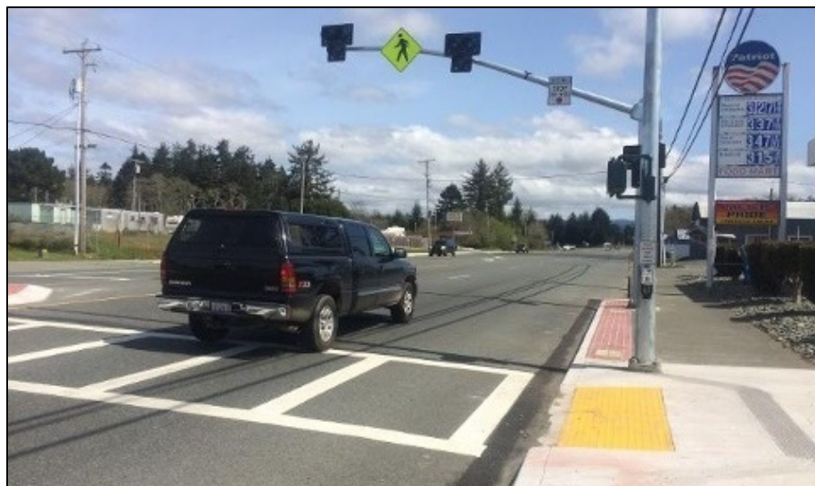
Figure 6-46: HAWK beacon on Highway 101 in Crescent City
