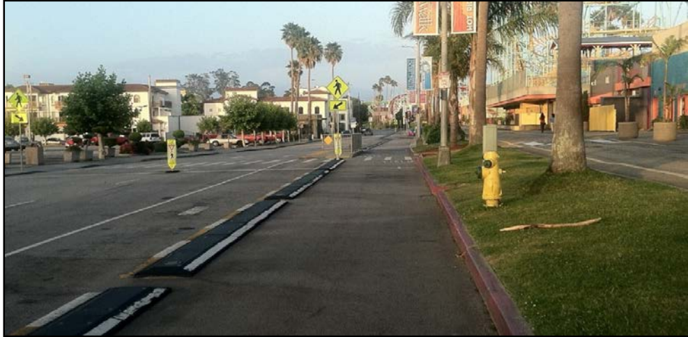
Figure 6-37: Separated bicycle lane in Santa Cruz, California
