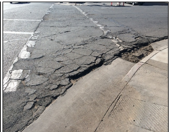
Figure 4-7: Poor crosswalk condition around Holt Park
