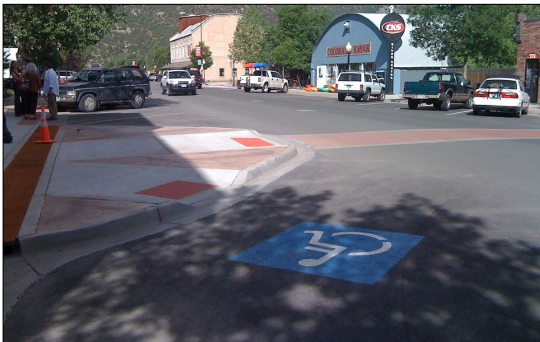
Figure 6-16: Curb extensions in Colorado
