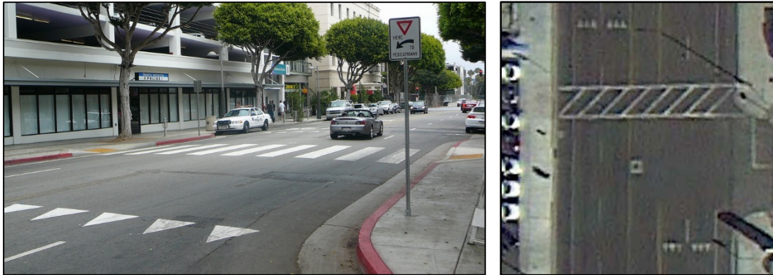
Figure 6-29: Advance yield markings in Santa Monica (left) and Bishop along SR 395 (right)
