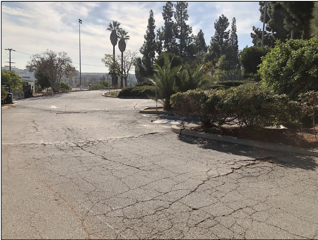
Figure 14. Photograph of cracked and buckled asphalt in parking lot on the 1111 Sunset Project property, view to the south.
