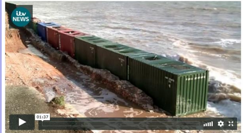
Shipping containers provide temporary flood defences at Dawlish
