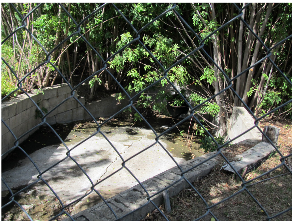
Photo 2. Storm drain outlet at northwestern portion of site that disperses into the site's drainage. Facing upstream.
