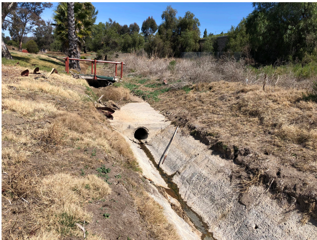
Photo 4. Site drainage transitioning from earthen bottom to concrete lined in central-east portion of site. Facing upstream.
