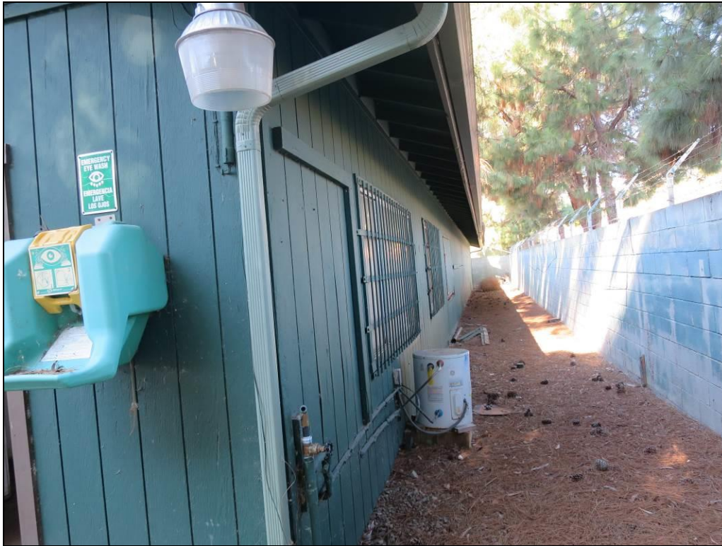
Figure 4: Northeast elevation of structure facing northwest. (photograph by IS Architecture 2017)
