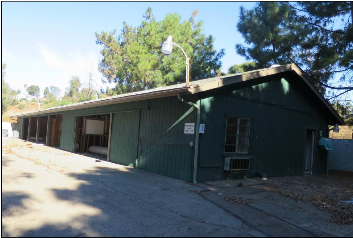
Figure 1: View of structure facing north. (photograph by IS Architecture 2017)
