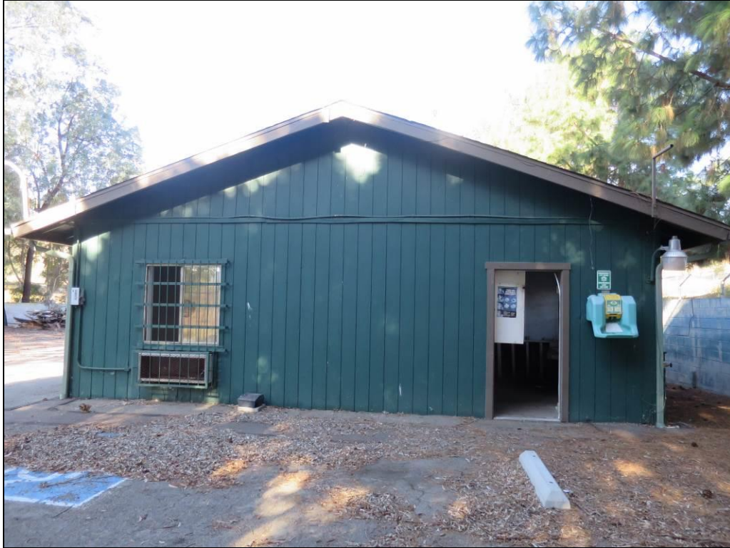
Figure 2: Southeast elevation of structure facing northwest. (photograph by IS Architecture 2017)
