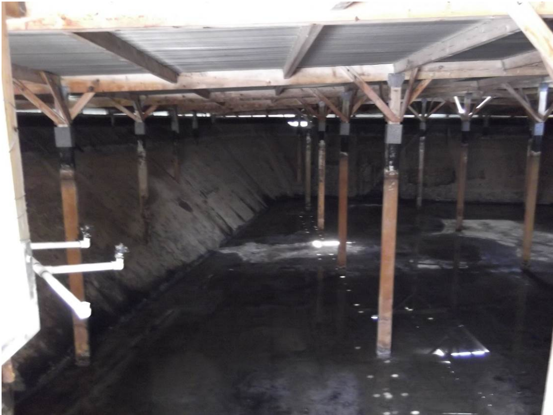
Figure 65. Interior of reservoir looking at wooden roofing support beams and struts. Looking east from the embankment stairway near the northwest corner.
