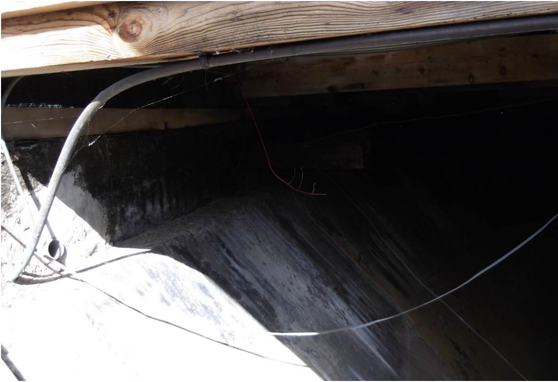
Figure 63. Raised curb perimeter foundation around the outside of the La Jolla Exchange Place Reservoir. Looking north at the northwest corner of the embankment stairs.
