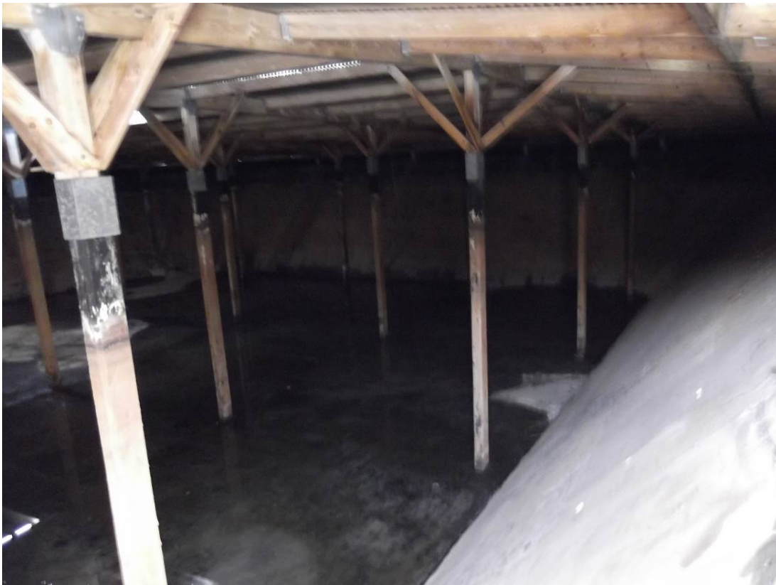
Figure 64. Interior of reservoir looking at wooden roofing support beams and struts. Looking south at the southwest corner from the embankment stairway.
