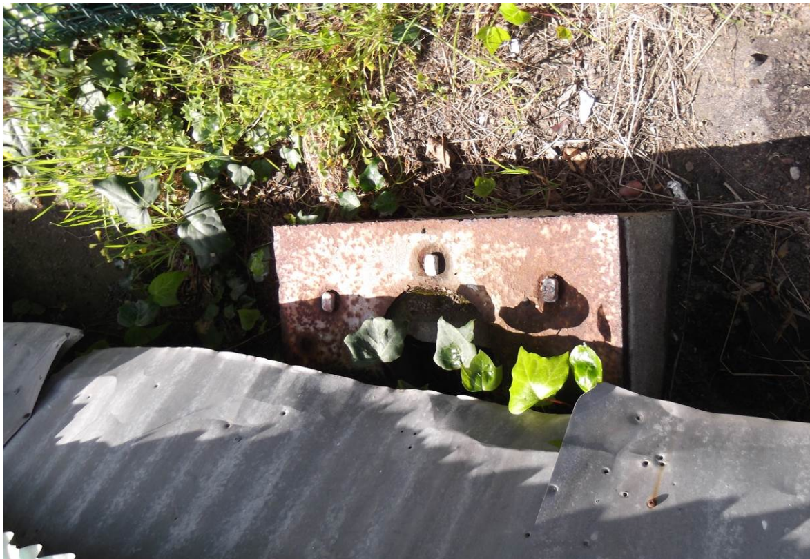
Figure 58. View of steel and concrete anchor block adjacent to the raised concrete perimeter foundation curb, located on the west side near the northwest corner.
