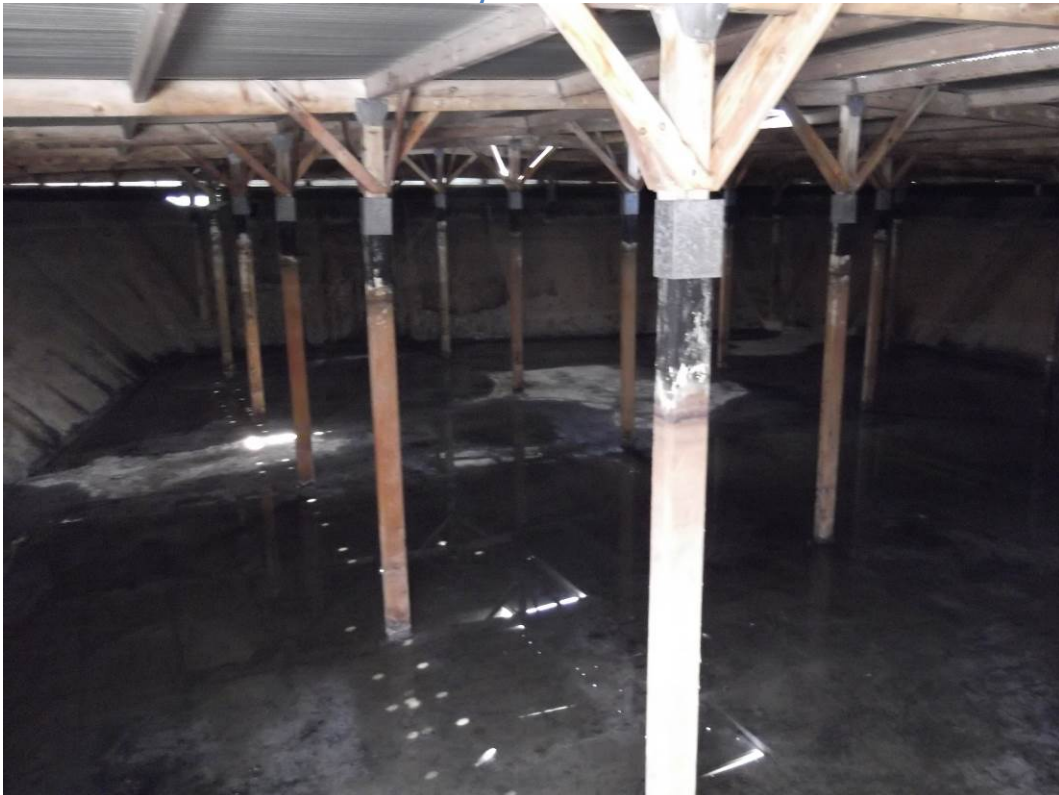
Figure 66. Interior of reservoir looking at wooden roofing support beams and struts. Looking southeast from the embankment stairway near the northwest corner.
