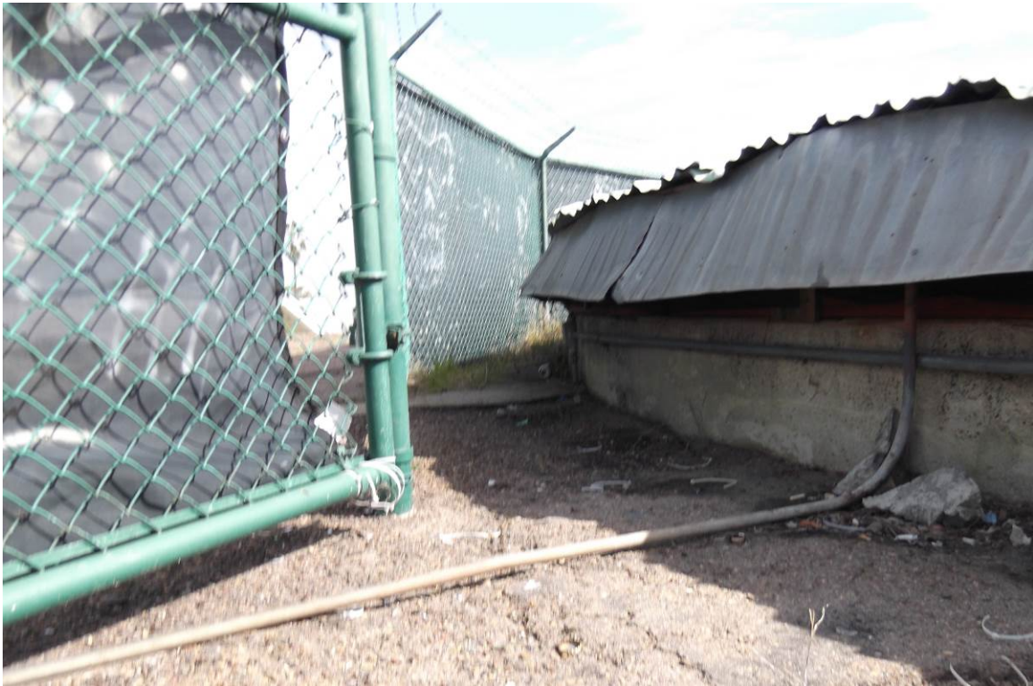
Figure 57. View of galvanized sheet metal skirting of La Jolla Exchange Place Reservoir above raised concrete perimeter foundation curb, looking west at the northwest corner.
