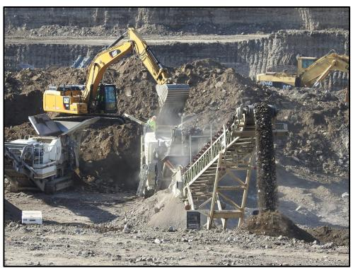
**2018 January** – Southeast Pit (Area 3S). Crushing and production of blended rubble fill. View to west.
