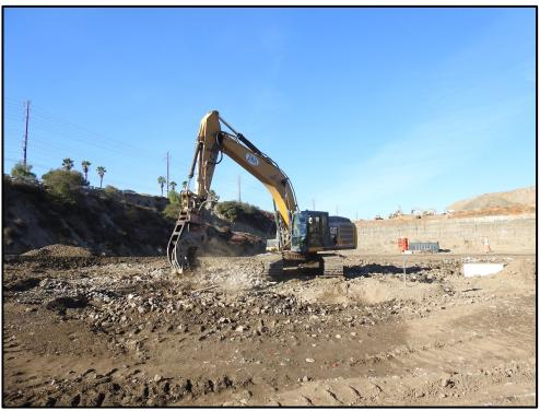
**2017 November** – Southeast Pit (Area 3S). Pulverization of oversized inert debris material. Settlement monument SM300 at right. New settlement monument SM310 with exposed base at far right. View to southwest.
