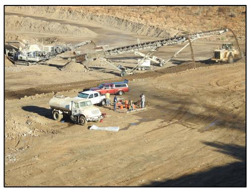
**2017 December** – Southeast Pit (Area 3S). Large-scale bulk density testing of blended rubble fill. In background, crushing of pulverized inert debris. View to northwest.
