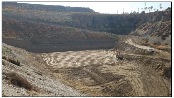
**2017 September** – West Pit (Area 1). Overview of exposed bottom in preparation for placement of engineered fill. View to east.
