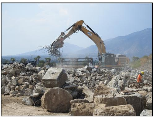
**2018 January** – South-Central Area (Area 2S). Removal of steel from inert debris. Large-scale field sieve in background. View to west.
