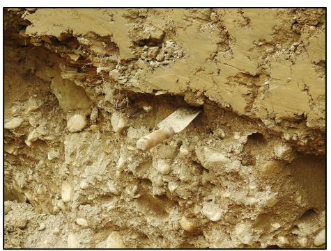
**2017** August – West Pit (Area 1). Geologic characterization of West Pit bottom materials. Trowel is stuck into side wall at contact of previously-placed silt and clay wash products and the underlying native sands and gravels. The wash products were removed in preparation for placement of engineered fill.
