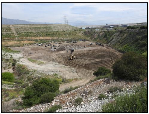
**2017 April** – Southeast Pit (Area 3S). Compaction of blended rubble fill. Area 3N surcharge fill in background. View to northeast.
