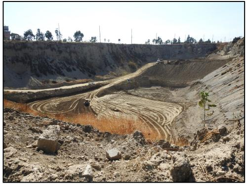
**2017 September** – West Pit (Area 1). Overview of new engineered fill pad. Removed and stockpiled wash products in background. View to southwest.
