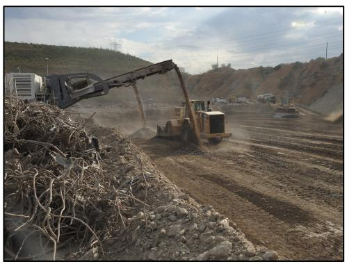
**2017** August – Southeast Pit (Area 3S). Crushing of pulverized inert debris, and compaction of blended rubble fill. View to northeast.
