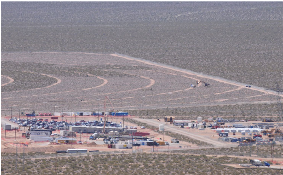
^Mowing and grubbing vegetation on the Ivanpah Solar Project, California
