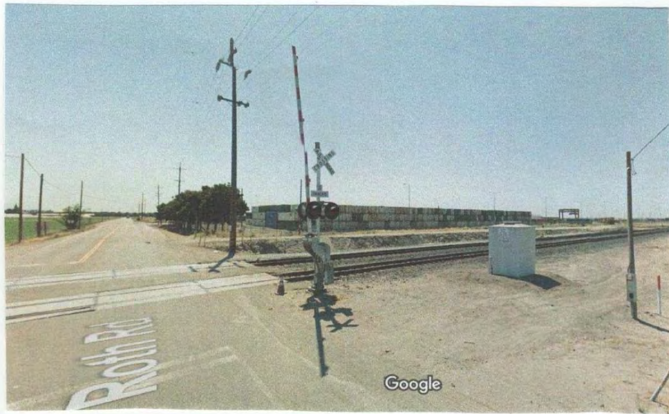
GRADE CROSSING SIGNALS AND GATE
