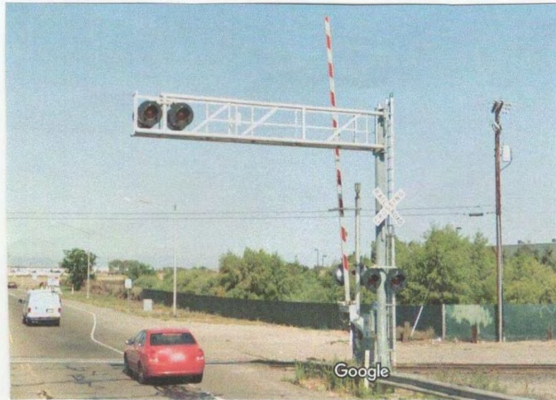
CANTILEVER SIGNAL
