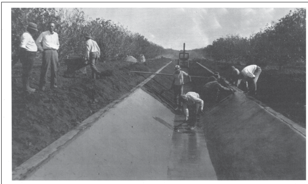
Figure 7. Concrete lining of unknown canal in 1930. (McSwain 105)
