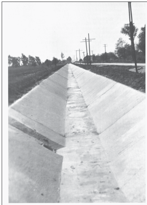
Figure 7. Concrete lining of unknown canal in 1930. (McSwain 105)
