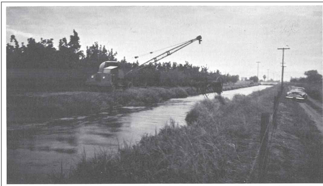
Figure 2. Crane cleaning weeds from an unknown canal in 1949. (McSwain 172)
