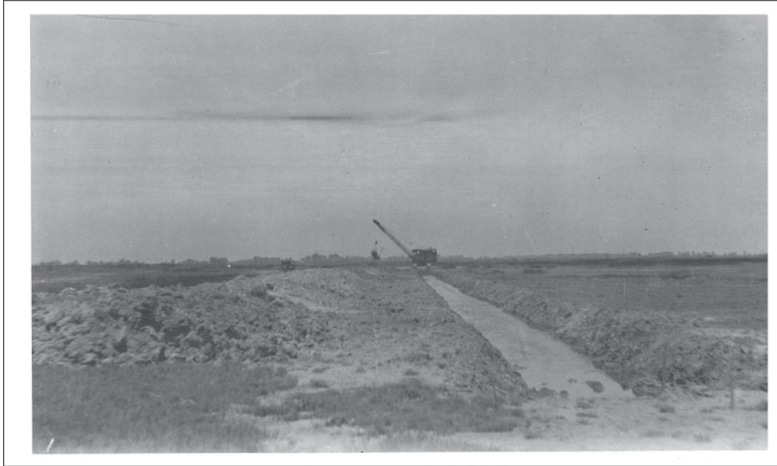
Figure 11. Dragline in 1929 digging a drainage ditch. (McSwain 95)
