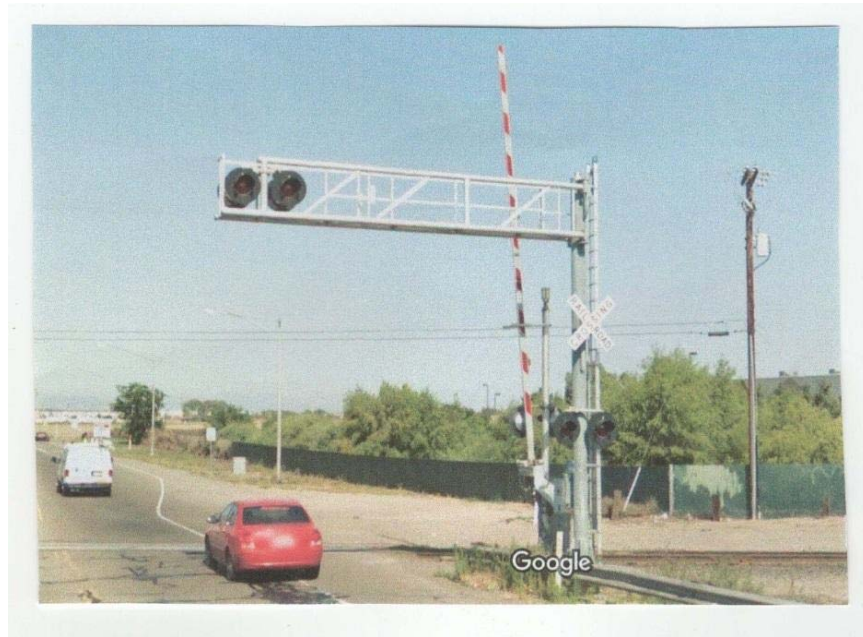
CANTILEVER SIGNAL
