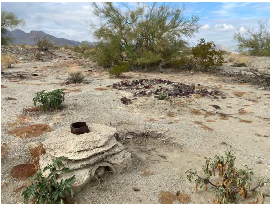
Subject Property; presumed water well (W4) cement base with steel pipe alongside apparent landfilling.
