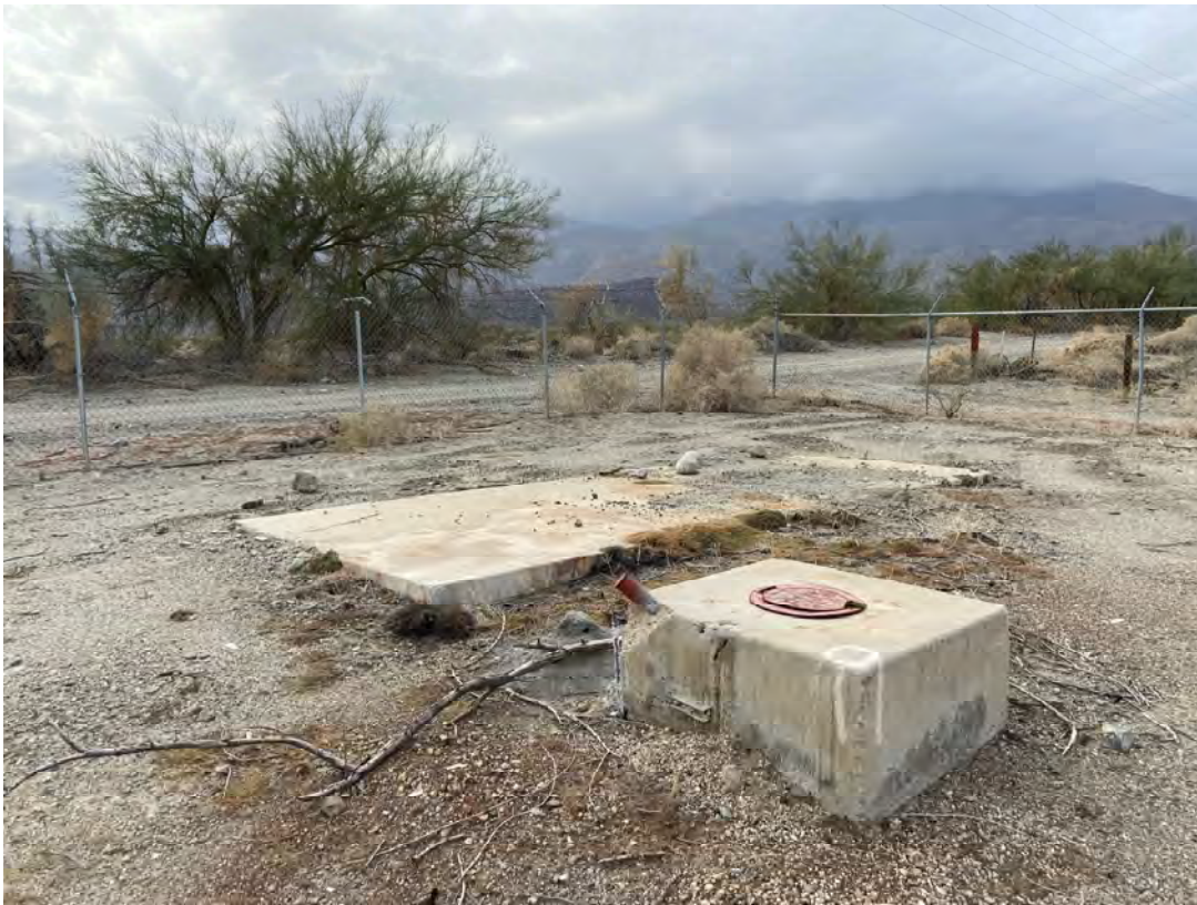
Subject Property; presumed agricultural water well (W3) with concrete slab surrounded with chain link fencing.
