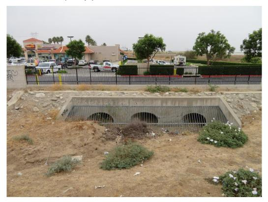
**Photograph 4:** Photo of the three 6-foot concrete culverts Drainage 1 discharges into located along the eastern boundary of the project site.
