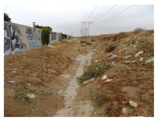
**Photograph 3:** View of the 2-foot concrete lined v-ditch portion of Drainage 1 located along the eastern boundary of the project site.
