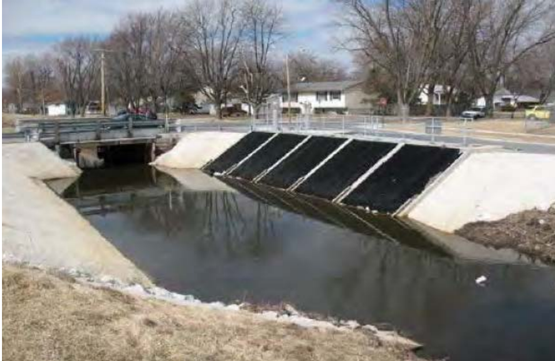
Figure G2-3. Typical intake structure with vertical bar trash rack
