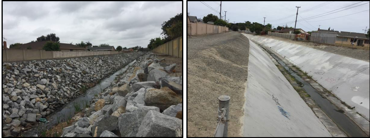
Typical existing trapezoidal channels. The picture on the left shows a typical existing riprap lined trapezoidal channel in the study area (before). On the right is a trapezoidal channel lined with concrete to improve conveyance efficiency (after).
