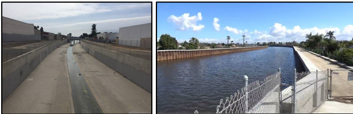
Examples of channel reaches with rectangular cross-sectional geometry to increase capacity and improve conveyance efficiency. On the left is a typical concrete lined rectangular channel. On the right is a soft bottom rectangular channel reach constructed using steel sheet pile walls.
