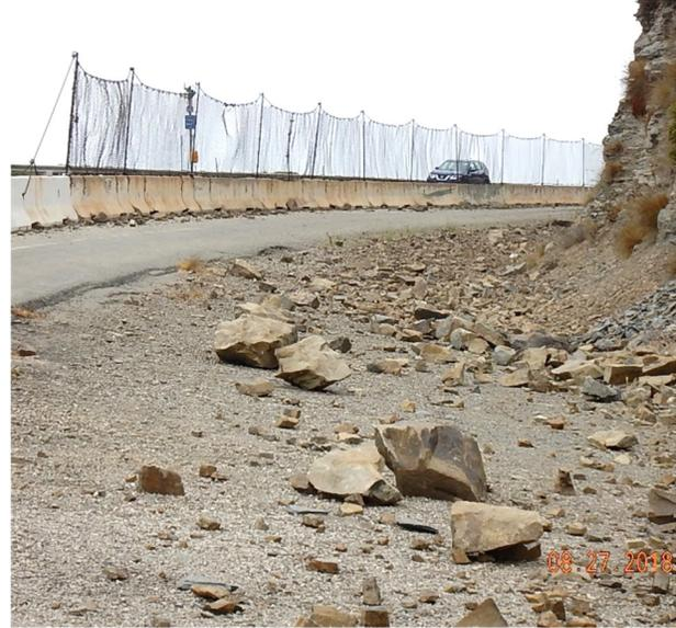
**Figure 1-17: Rocks lying within the shoulder blocked from vehicle access with k-rail and fencing. Photo taken on August 27, 2018.**
