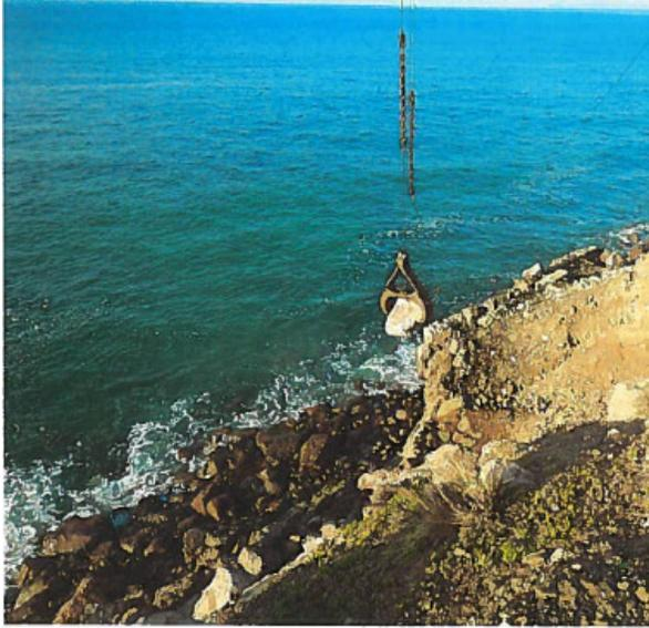
**Figure 1-6: Crane placing 8-ton boulder at the toe of the slope at PM 4.0. Photo time stamped on 02/02/2015.**
