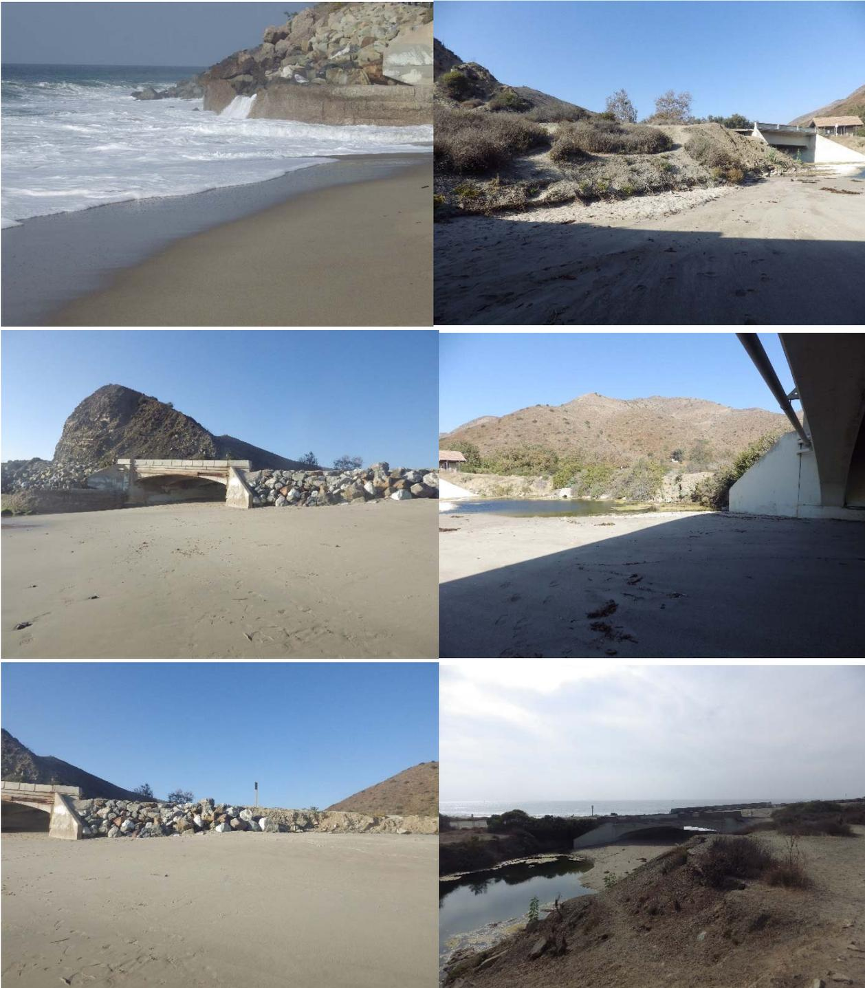
**Figure A-1-5: Site conditions at Big Sycamore Creek Bridge. The three photos on the left are from the beach and the three on the right are from the north side of the bridge. Photos taken October 2017. The loss of seawall height is evident in the top left photos where the wave runup back wash is spilling over the wall. The bottom left photo shows the rock revetment next to the bridge and eroding slope immediately beyond the protective rock.**
