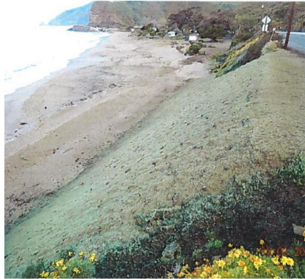
**Figure 1-8: Fill slope at PM 4.2 was repaired in-kind without rock slope protection at the toe of the slope. Photo taken on 03/02/2015.**
