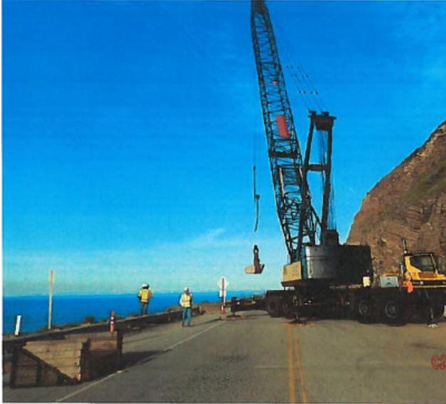
**Figure 1-5: Construction of 8-ton boulder placement onto the fill slope at PM 4.0. Photo taken on 02/02/2015.**
