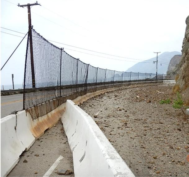
**Figure 1-16: K-rail and fencing deployed within the project area. Photo taken on August 27, 2018.**
