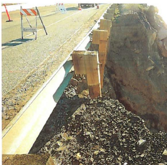
**Figure 1-4: Guardrail at PM 4.0 shown hanging off the roadway due to severe slope erosion. Photo taken on 01/14/2015.**
