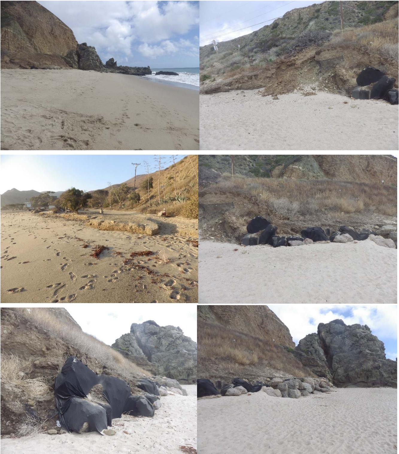
Figure A-1-3: Photos at southeast end of beach from March 2018 showing: top left entire beach with erosion escarpment in left of photo, middle left (this photo from Oct. 2017) former location of life guard structure lost during Hurricane Marie, bottom left exposed geotextile and mesh in erosion escarpment. Top to bottom on right is a pan of the erosion escarpment, toe protection rock and headland.
