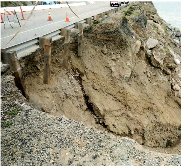
**Figure 1-3: Fill slope eroded at PM 4.0 with guardrail hanging. Photo taken on 01/29/2015.**
