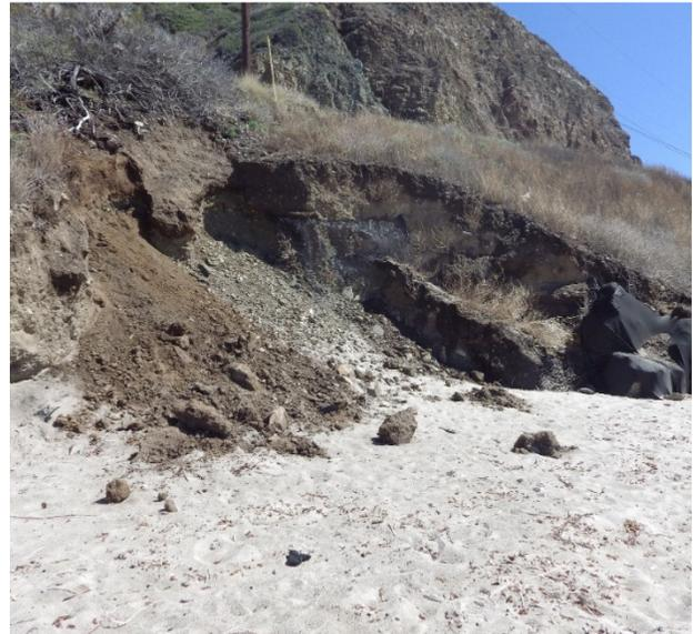
**Figure 1-12: Slope at PM 4.2 showing erosion failure. Photo taken on March 15, 2018.**
