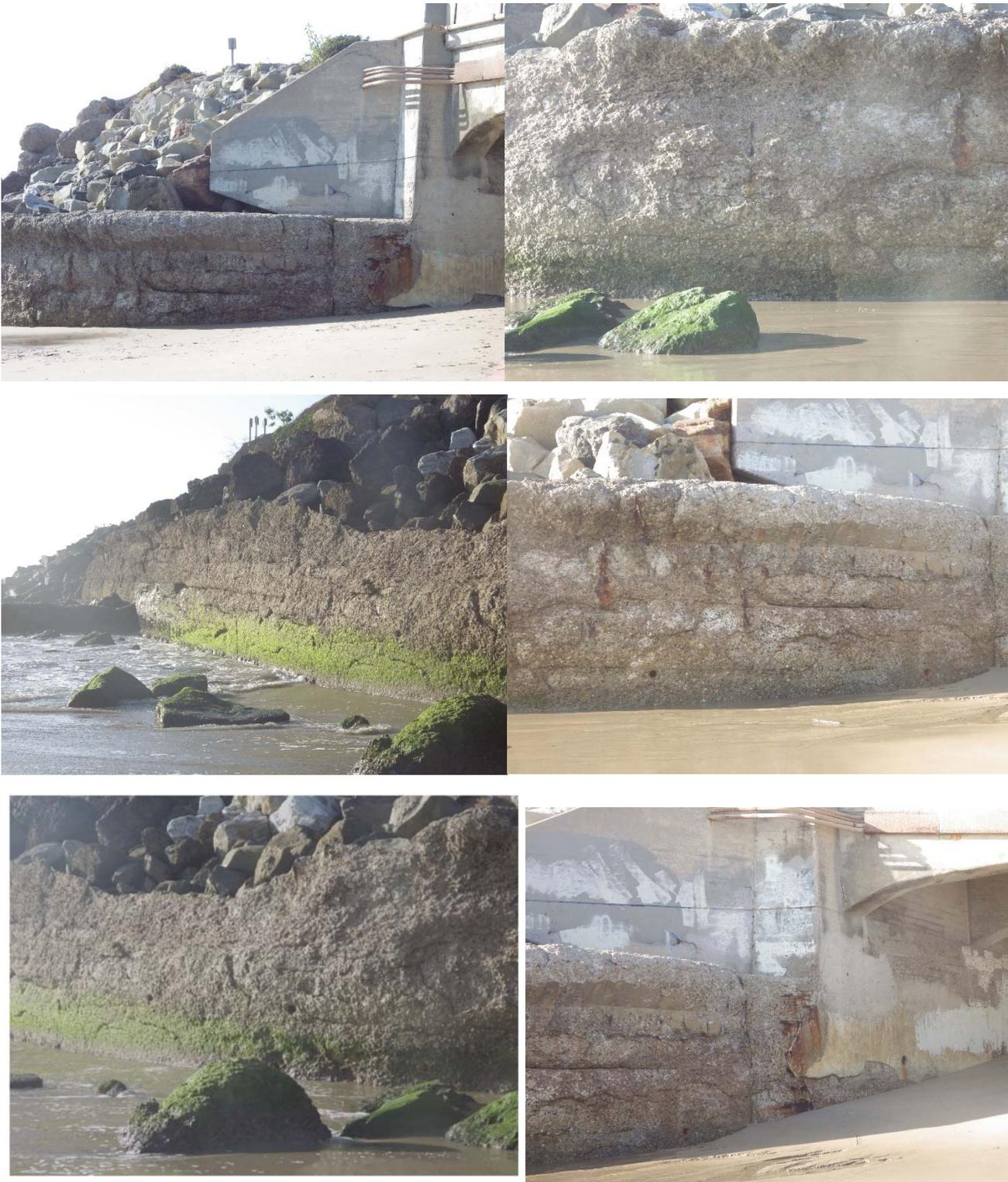
Figure A-1-7: Site conditions at the seawall and bridge abutment in October 2017. Top left is abutment and seawall with utilities that cross the bridge. Middle left to bottom left then top right to bottom is a pan from offshore to the bridge of the seawall. The low part of the seawall is shown at the bottom left. The deterioration at the interface between the bridge abutment and seawall is evident in the bottom right photo.
