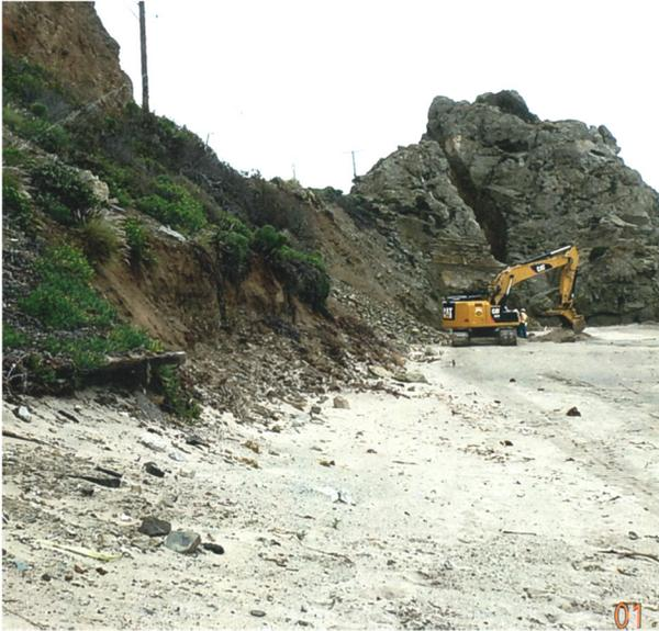
**Figure 1-7: Slope erosion at PM 4.2 after Hurricane Marie in August 2014 and additional storms in December 2014. Photo taken on 01/29/2015.**
