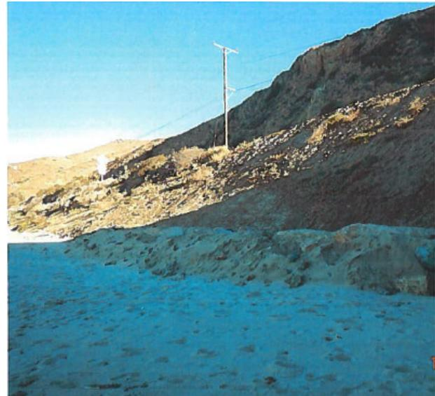
**Figure 1-10: Rock slope protection is constructed at the toe of the slope after high surf causes the fill slope to erode. Photo taken on 12/17/2015.**
