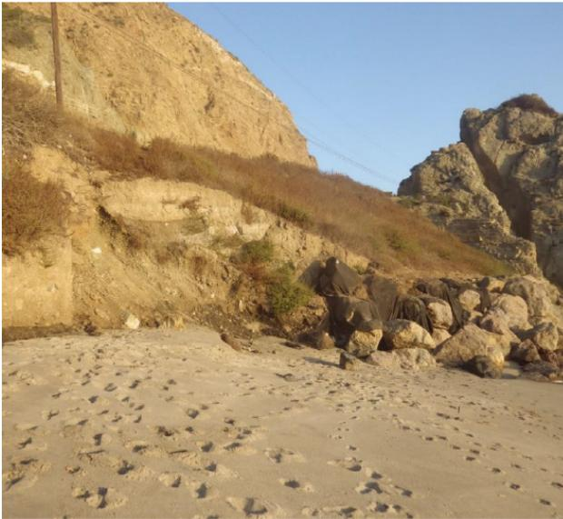
**Figure 1-11: Slope on PM 4.2 in October 2017. Slope has eroded to meet the rock slope protection wall at the toe of the slope.**
