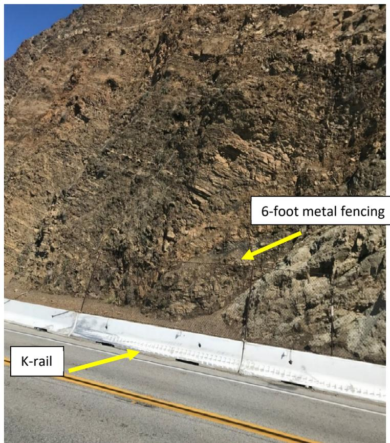
**Figure 1-15: Access on the shoulder of northbound PCH through the project area is blocked with K-rail and metal fencing.**
