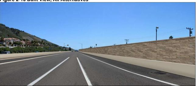
If it were constructed, an 8-foot-tall soundwall would be placed along the edge of the southbound freeway shoulder, possibly fronted by a concrete safety barrier. Existing vegetation between US 101 and Shell Beach Road would be removed to accommodate the part-time travel lane, and the existing concrete barrier in the median would be replaced with a taller style.
