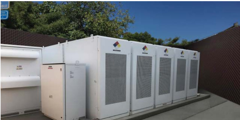
Exhibit 6-5: Example of battery storage
