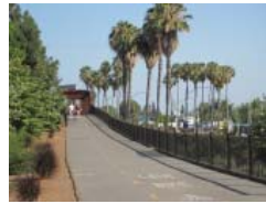
Class I: Shared-Use Path Provides a completely separated right-of-way for the exclusive use of bicyclists and pedestrians
