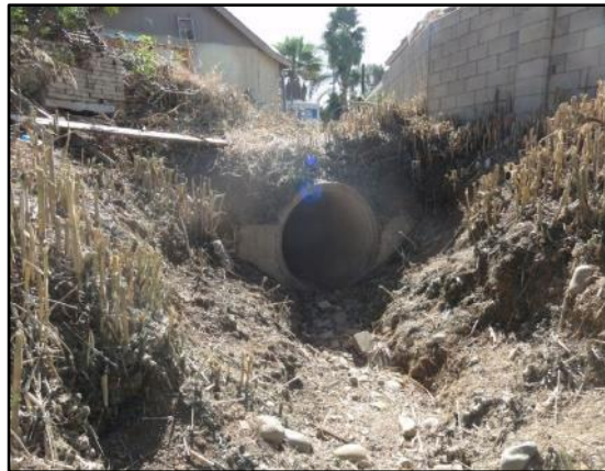
12. Lobrico 1, Reach 1: End of Lobrico 1 at inlet of 48-inch RCP beneath Jamacha Road, looking southwest (November 2016).
