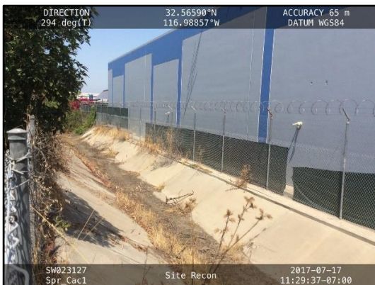
3. Cactus 2: Sediment deposition in basin.
