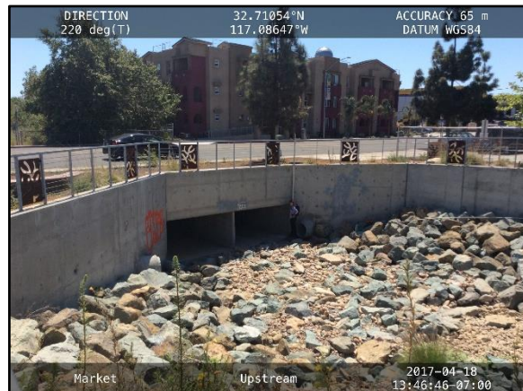
4. Euclid 1: Double box culvert inlet at Market Street.
