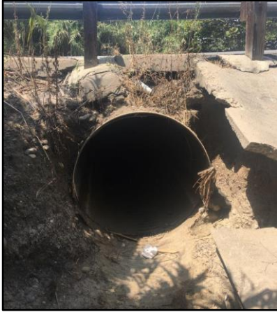
3. Jamacha 2: Upstream of the Cadman Street culvert (54-inch-diameter corrugated metal pipe), facing west.
