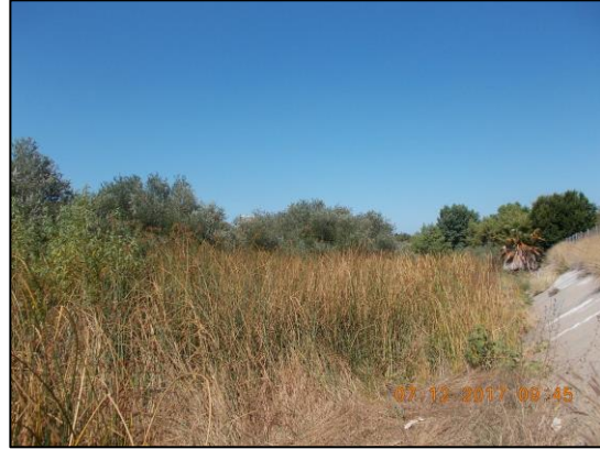
6. Alpha 1 (Reach 1): looking downstream, showing vegetation in the earthen channel bottom and the concrete right bank.
