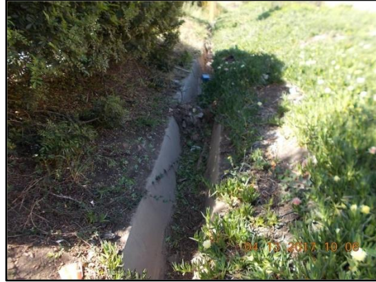
4. Outer 2: Looking downstream at debris/sediment and overhanging vegetation upstream of Outer 1 and Outer 2 junction.
