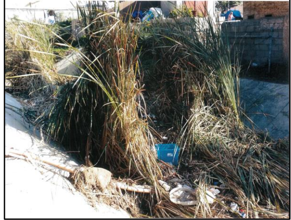
3. Via de La Bandola 1, Map 1: Looking upstream at dense vegetation and sediment/debris within channel.
