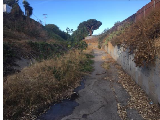
8. Solola 1: Looking downstream at accumulated sediment/debris in concrete channel. (November 2017)
