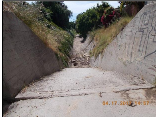
6. Solola 2 (Reach 1): Looking downstream at second drop structure and sediment accumulated at bottom of structure.
