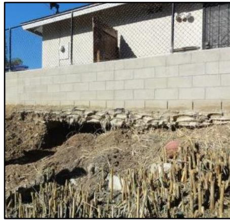
10. Lobrico 1, Reach 1: Scour hole underneath the private masonry wall on right channel bank, looking southwest (November 2016).
