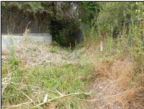
5. Lobrico 1, Reach 1: Dense vegetation present in channel and start of the 3-foot high private masonry wall along right bank, looking north (July 2019).
