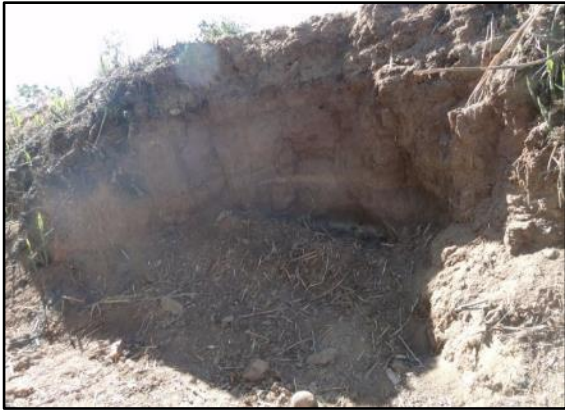
3. Lobrico 1, Reach 2: Erosion along right bank, at outlet of 48-inch RCP beneath Lisbon Street, looking southwest (November 2016).
