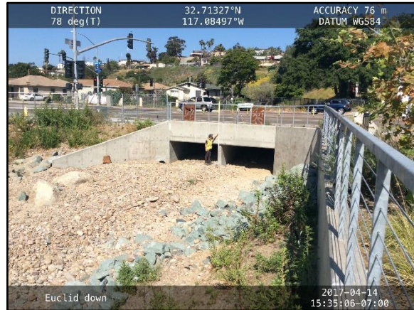
2. Euclid 1: Double box culvert outlet at Euclid Avenue.
