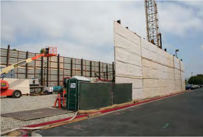
I-Beam & Acoustic Material 03
