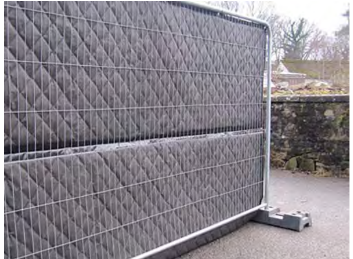
Temporary Fence & Acoustic Material 01
