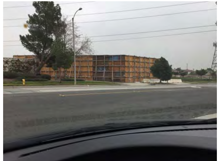
K-Rail Plywood & Acoustic Material
