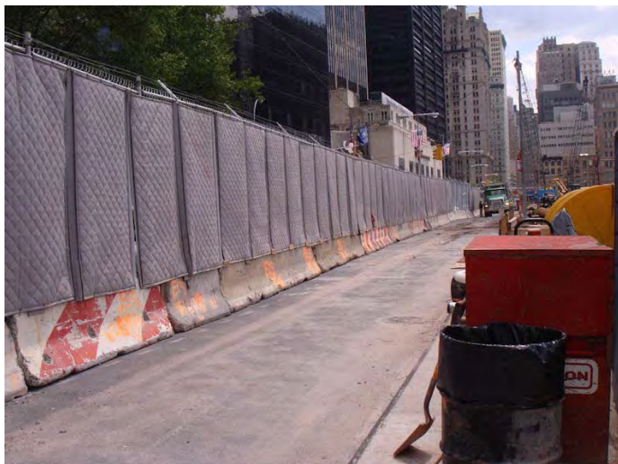
K-Rail Temporary Fence & Acoustic Material
