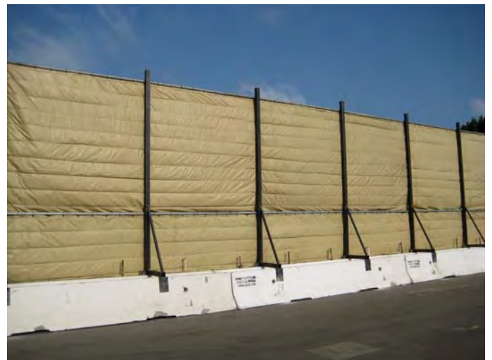
K-Rail-Mounted Acoustic Material 01
