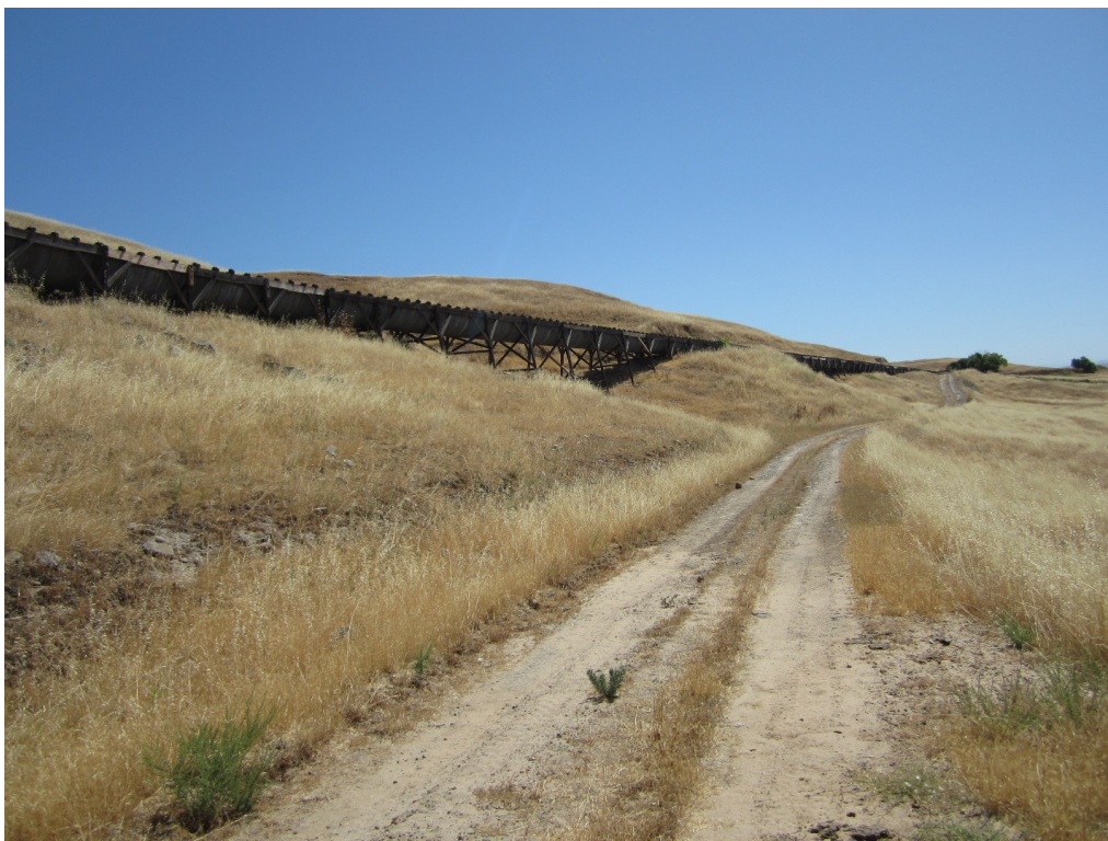
Photograph 3. Northside Canal, wooden flume segment, view east.
