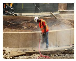
A worker breaks up concrete creating a cloud of silica dust.
