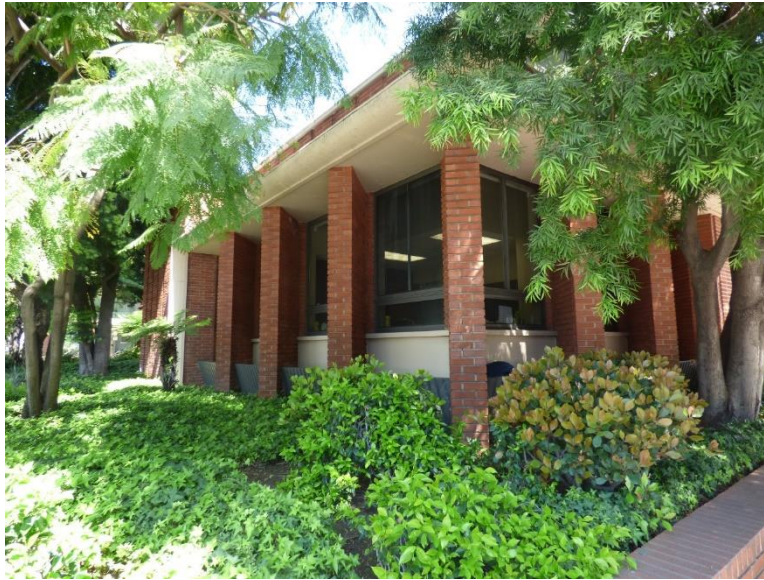
Figure 31 JWCI's Sunshades on the West Corner of the 1952 Addition, view east
