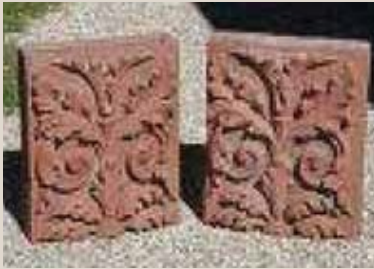
Cast and fired clay units, used as ornamentation.
