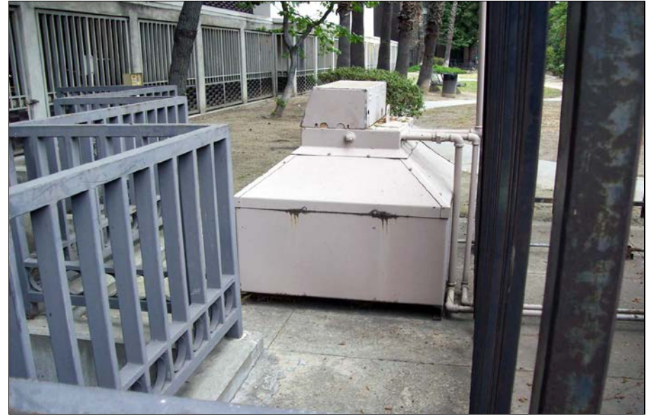
Photo 2: Day tank for generator.
