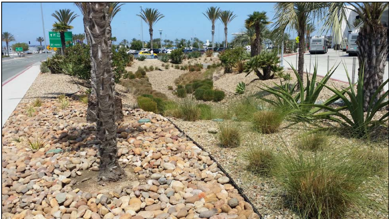
Photo 4. Another example of a maintained stormwater bioretention basin at SDIA.
