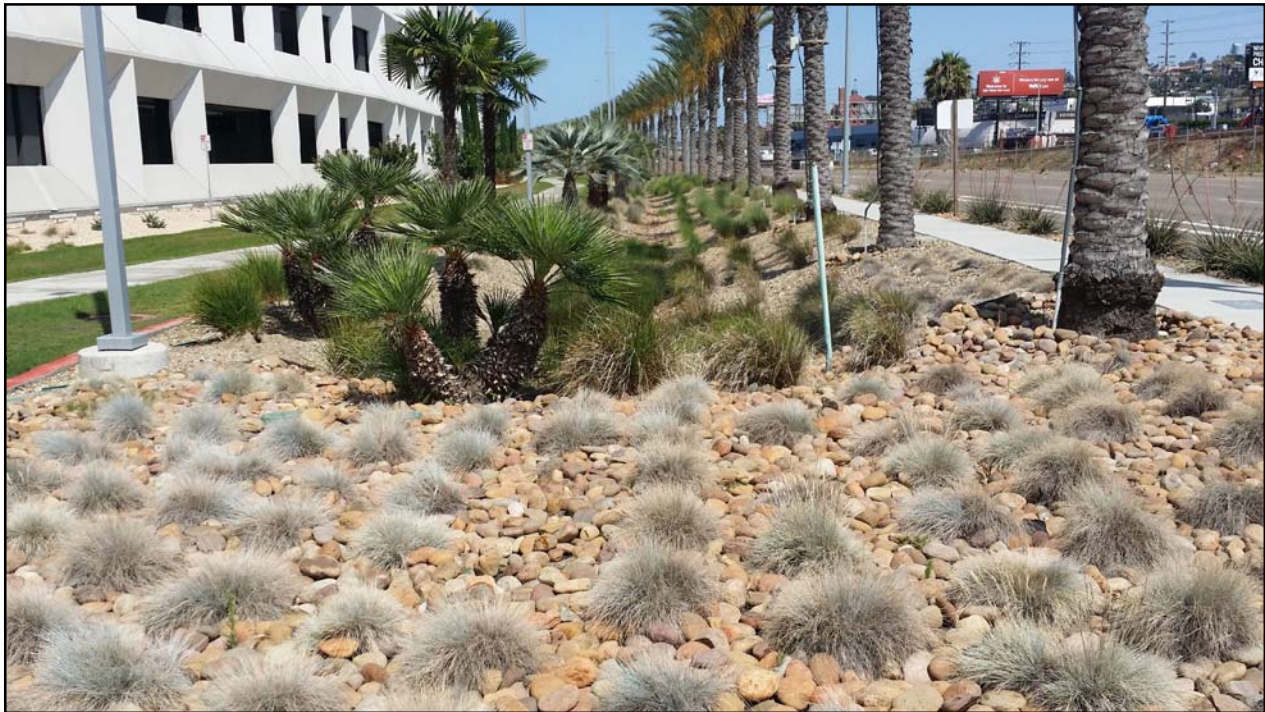
Photo 3. Example of a maintained stormwater bioretention basin at SDIA.
