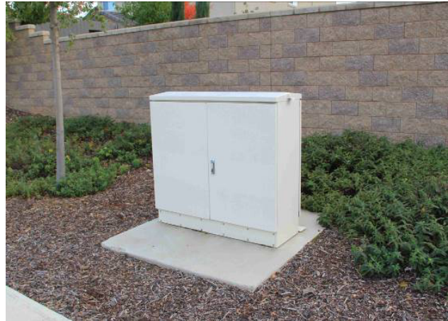
Figure 18 – AT&T Primary Flex Point
