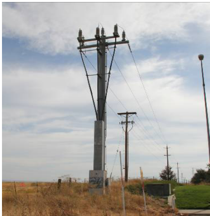
Figure 7 – Roseville Electric 60kV Riser
