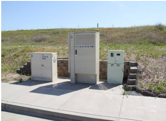
Figure 20 – AT&T Remote Terminal Cabinet
