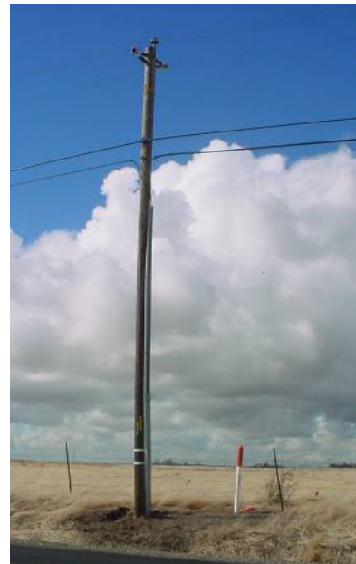
Figure 24 – Sprint Fiber Line on PG&E Poles
