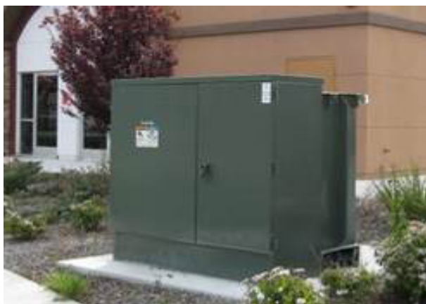
Figure 14 – Three Phase Transformer
