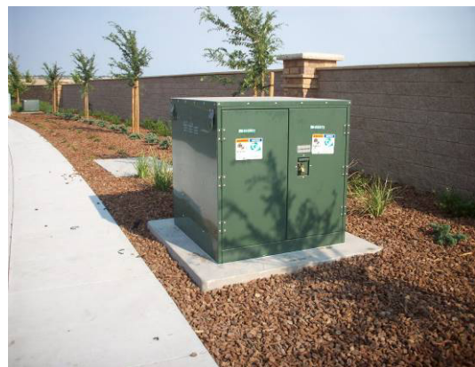
Figure 12 – Pad Mounted Interrupter
