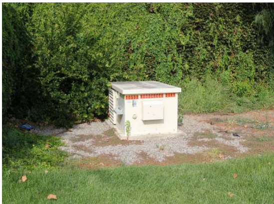
Figure 11 – AT&T Controlled Environment Vault
