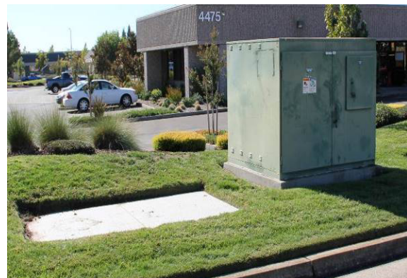
Figure 15 – Capacitor Bank w/ #7 Box
