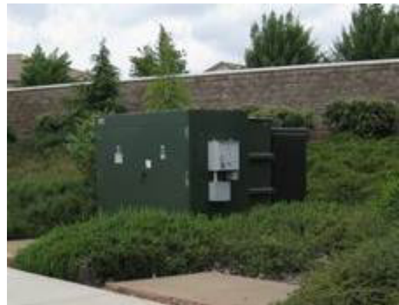
Figure 17 – 21kV to 12kV Auto-bank
