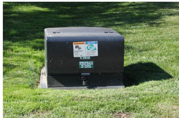
Figure 13 – Single Phase Transformer
