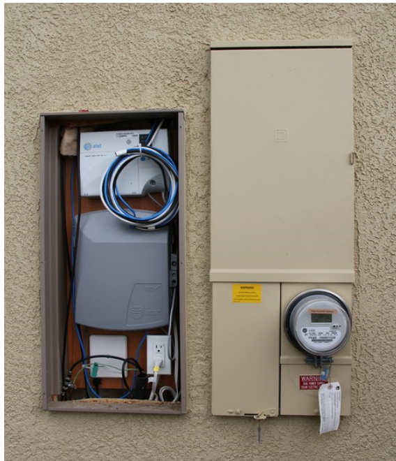
Figure 19 – Optical Network Terminal adjacent to an Electric Meter Panel
