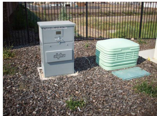
Figure 22 – Cable TV Fiber Node & Power Supply
