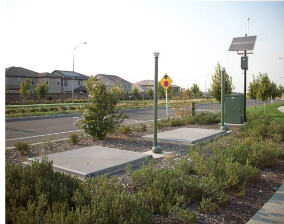
Figure 10 – PG&E Gas Regulator Station w/SCADA Controller– Westbrook Blvd.
