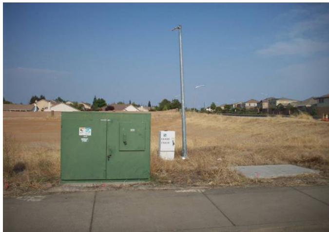
Figure 16 – Pad Mount Capacitor Bank with SCADA Controller & Antenna for a Subsurface Switch
