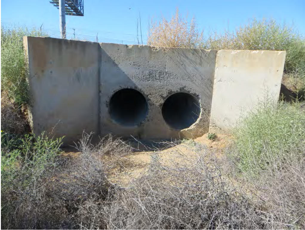
Photograph 9: Facing west (upstream) at two 36-inch culverts at the western end of Drainage 2. Interstate 215 is in the background.
