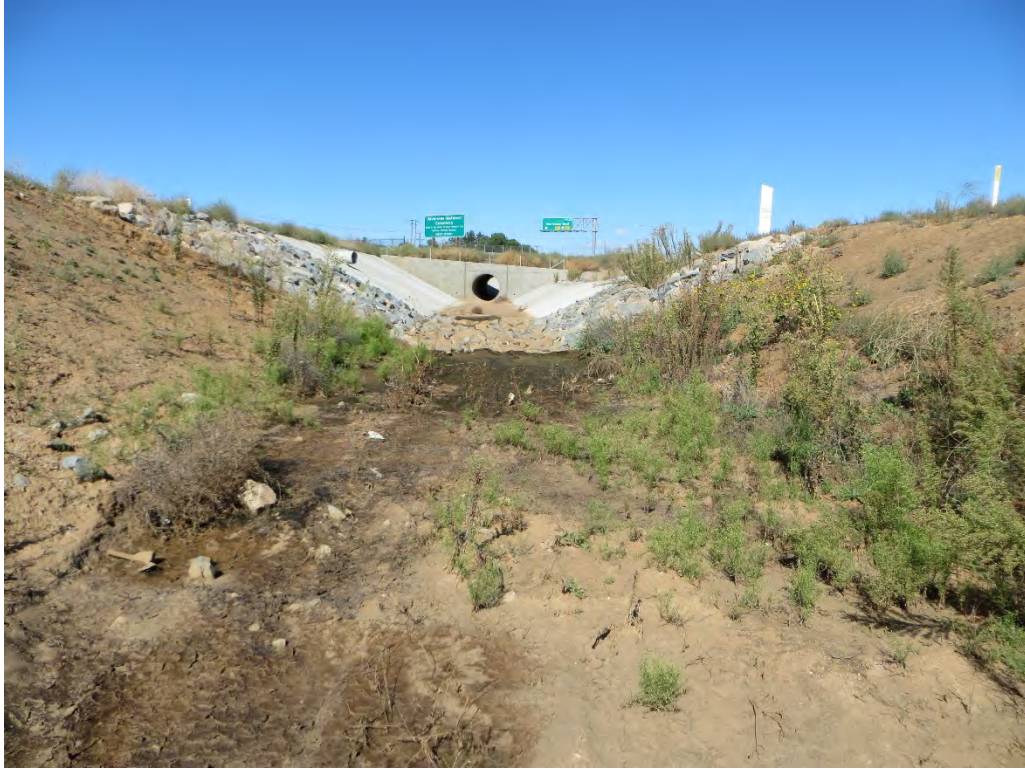
Photograph 1: Facing the northwest terminus of the project site (upstream) from within Drainage 1. Drainage 1 is lined with riprap within the project boundaries, but then becomes earthen. Outside of the project boundaries, the drainage is lined with cement.
