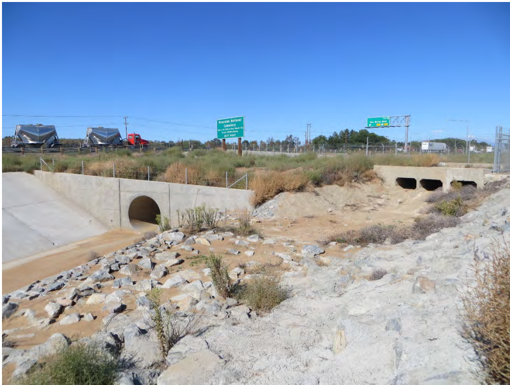
Photograph 14: Facing northwest at the confluence of Drainages 1 (left) and 4 (right). Drainage 4 sheetflows over the top of Drainage 1.
