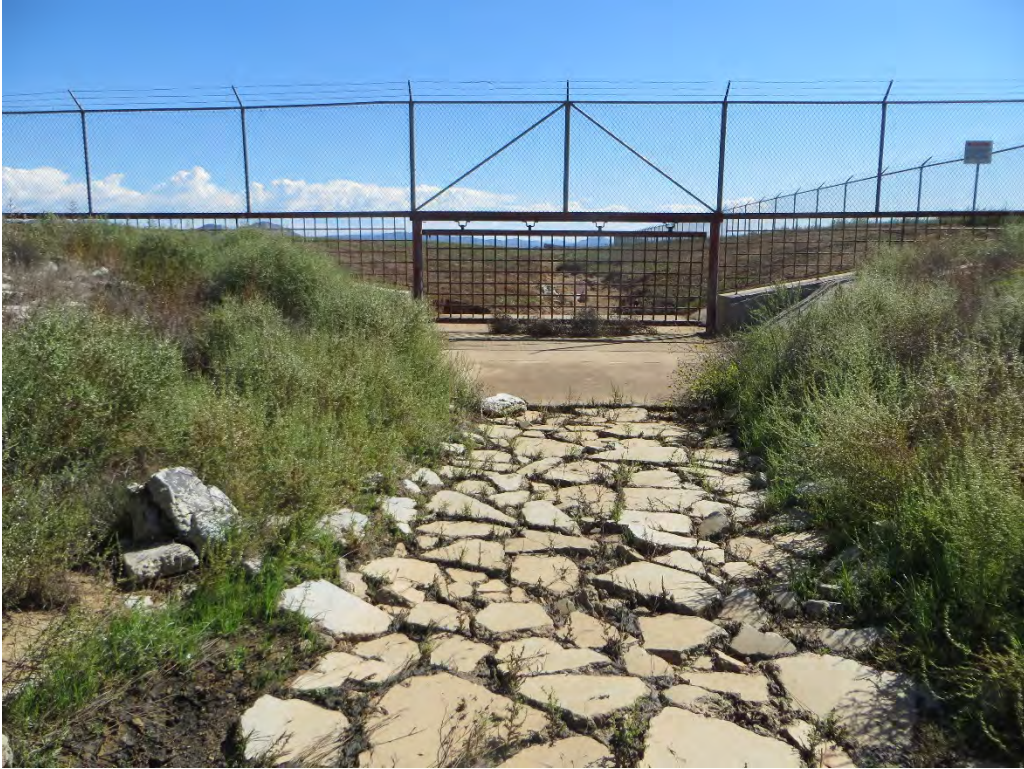
Photograph 7: Facing southeast (downstream) at the southern terminus of Drainage 1 within the project site. This end of the drainage is lined with rock and then with cement before the fence.
