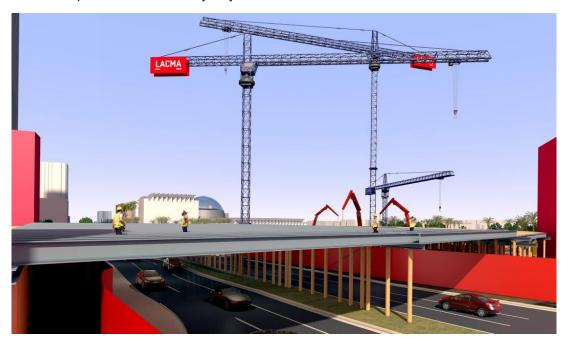
The falsework will be composed of steel and wood elements that will span Wilshire Blvd with temporary intermediate supports (columns) in the existing median of Wilshire Blvd. These temporary supports and adjacent protective elements will be robust enough to withstand vehicle impacts. These supports will require removal of the west bound left turn lane from Wilshire Blvd at Spaulding Avenue during falsework erection.
