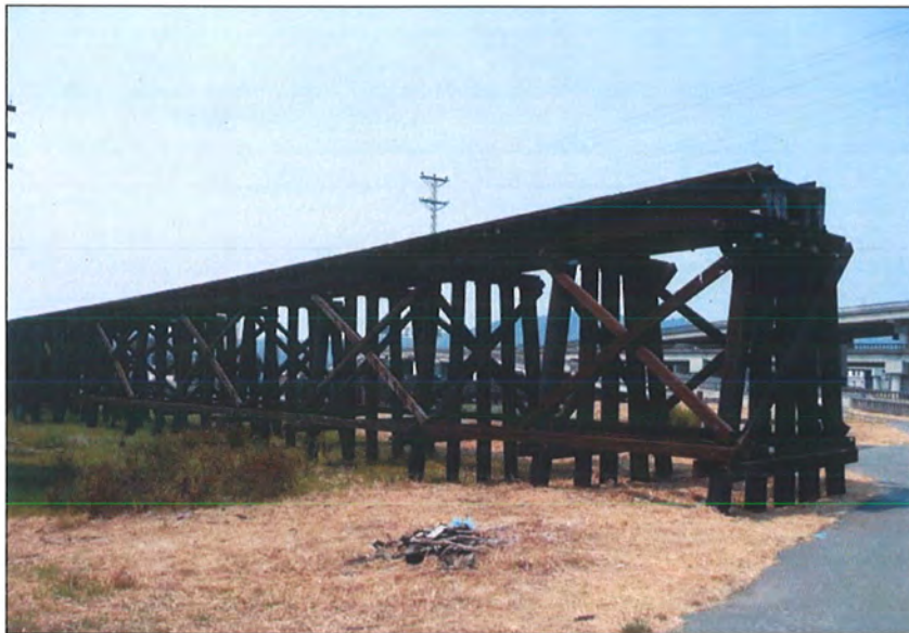
Photograph 3: View of trestle showing "X" braces, camera facing southwest.
