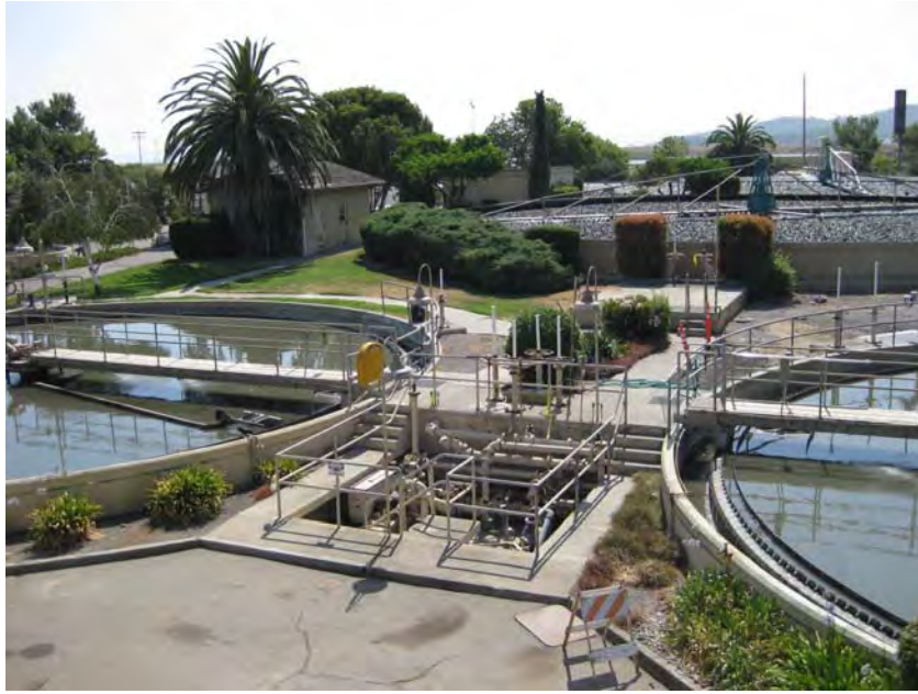
Clarifier #1 and #2 with Sludge Scum Pit in the center, and Primary and Secondary Biofilters in the background.
