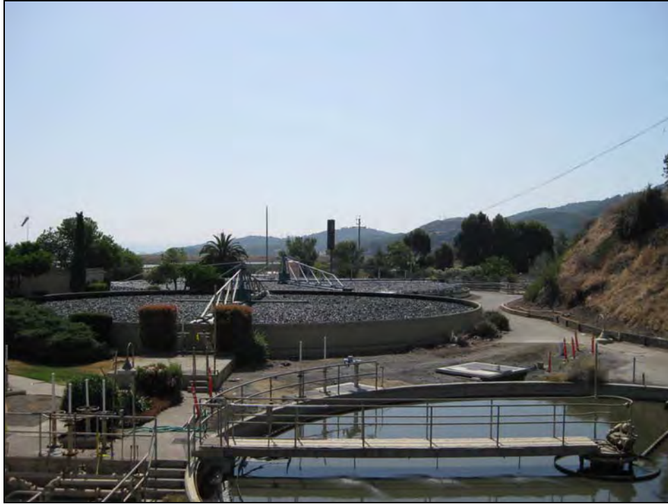
Figure 4. The Clarifier # 2 with Primary and Secondary Biofilters behind at the LGVSD Wastewater Treatment Plant.
