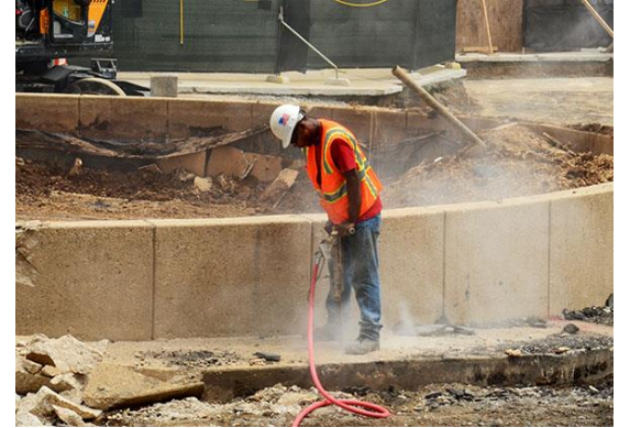
A worker breaks up concrete creating a cloud of silica dust.
