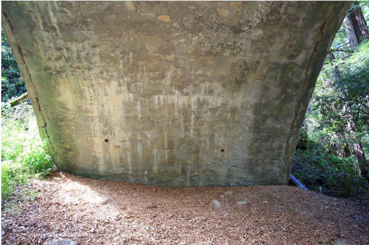
Figure 1 Picture of concrete arch looking westward at the western abutment. The two bore holes can be seen here where coring of the bridge was done for the 2011 in-depth geotechnical investigation (Petska, 2011).
