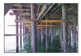
("stringers"). At the south end of the Wharf, horizontal members (ledgers) were installed at elevation 9 ft. MLLW (12 feet below top of pile) to provide lateral bracing to the piles, which are longer due to water depth at the end. The photo above shows a representative view of the Wharf pile and bent components. On average, 10 to 30 piles are replaced each year. Two inches of asphalt paving overlays the Wharf deck on roads and walkways.
