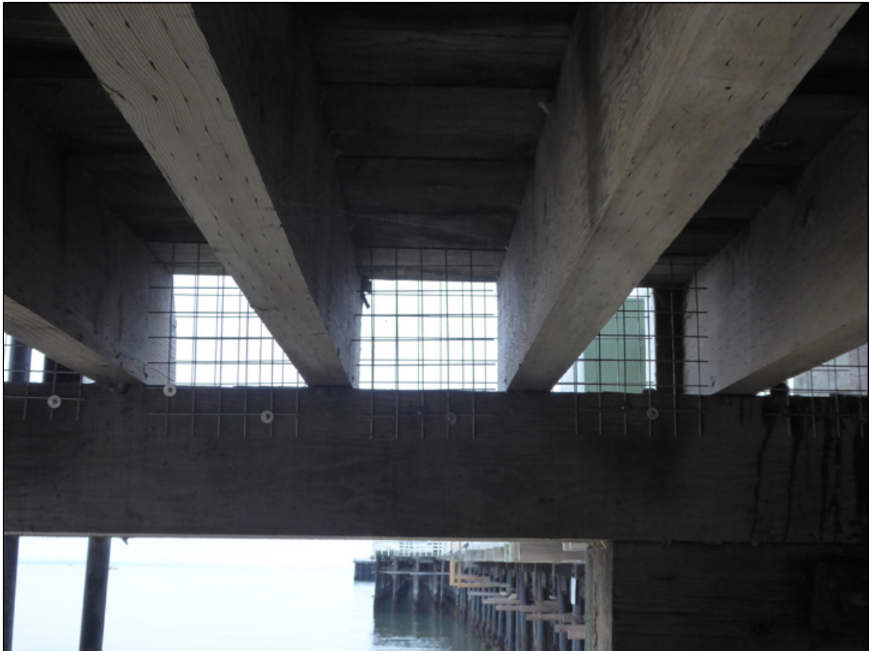
FIGURE 4. Pigeon Screening to Reduce Available Nesting Habitat
