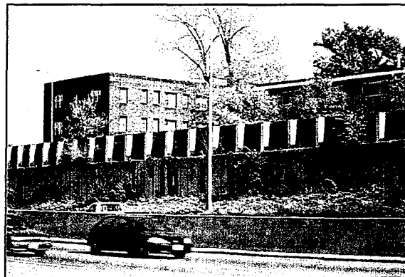
Figure 66. Combination cast-in-place retaining wall and noise wall (data base #329).
