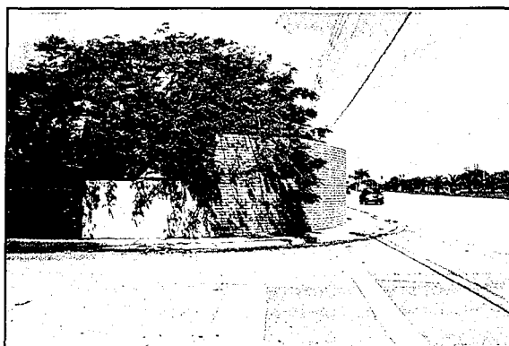
Figure 15. Barrier curved inward toward the community (data base #2617).
