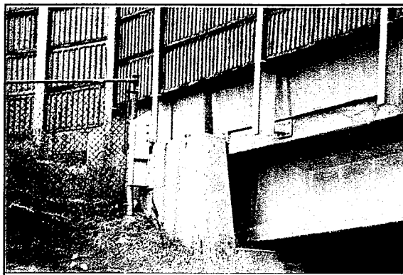
Figure 205. Expansion and contraction of barrier materials: connections between barriers (data base #463).
