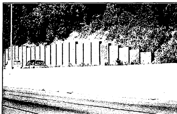
Figure 143. Barrier end treatment: buried into existing ground (data base #80).
