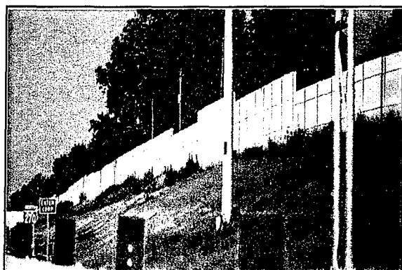
Figure 135. Vertical stepping of panels: irregular (data base #111).
