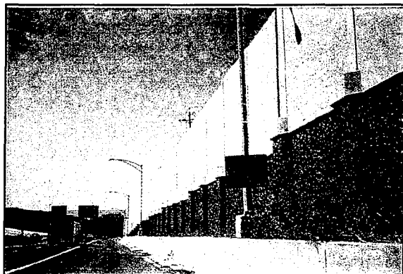
Figure 65. Combination cast-in-place retaining wall and noise wall (data base #5004).
