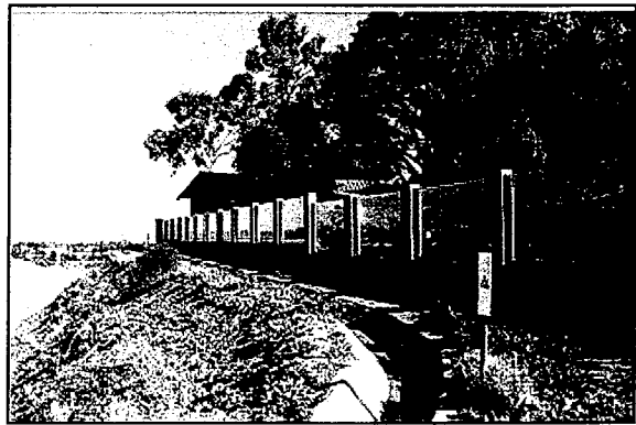
Figure 189. Drainage: water along a barrier (data base #984).
