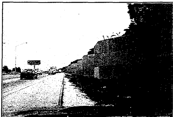
Figure 44. Precast free standing concrete noise wall (data base #1206).
