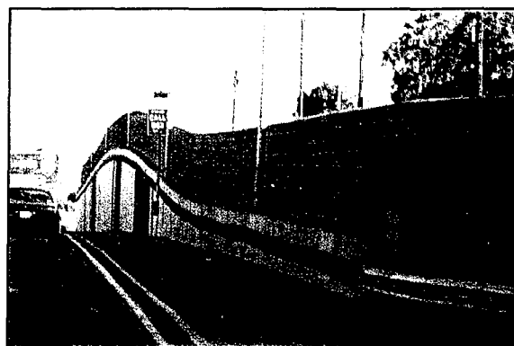
Figure 136. Vertical sloping of panels: smooth (data base #1839).
