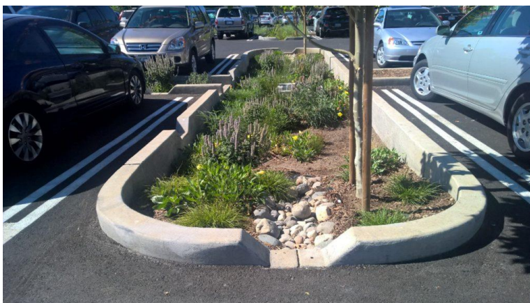
Figure 3: Curb Cut located in a Bioretention Facility
