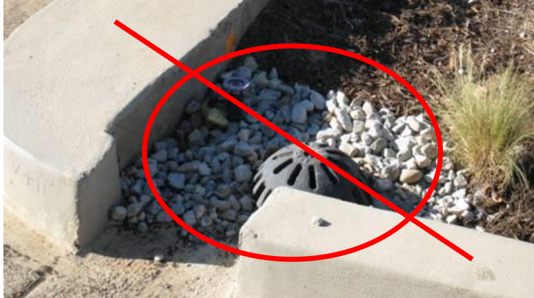
Figure 6: Incorrect Placement of an Overflow Inlet
