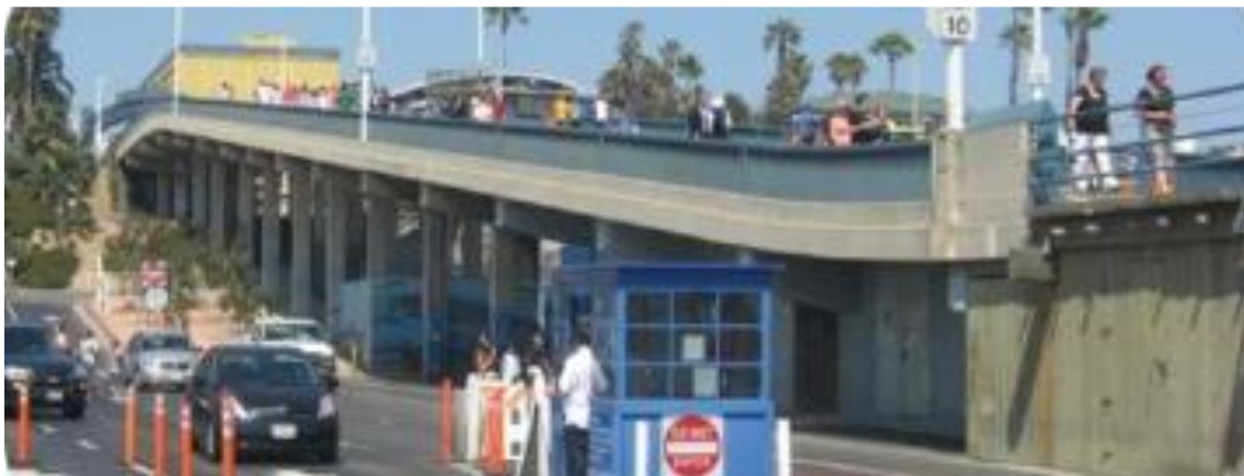
Photo 1-2. Steep Grade of the Santa Monica Pier Bridge
