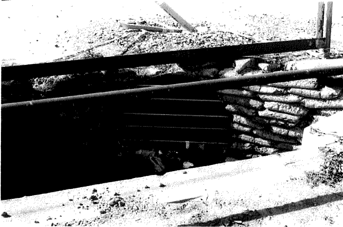
Photo 5: View of more modern "sac-crete" (concrete laid in sacks) headwall of culvert. This feature is located on the westernmost end of the drainage channel, and the culvert flows to the Burbank Western Flood Control Channel.
