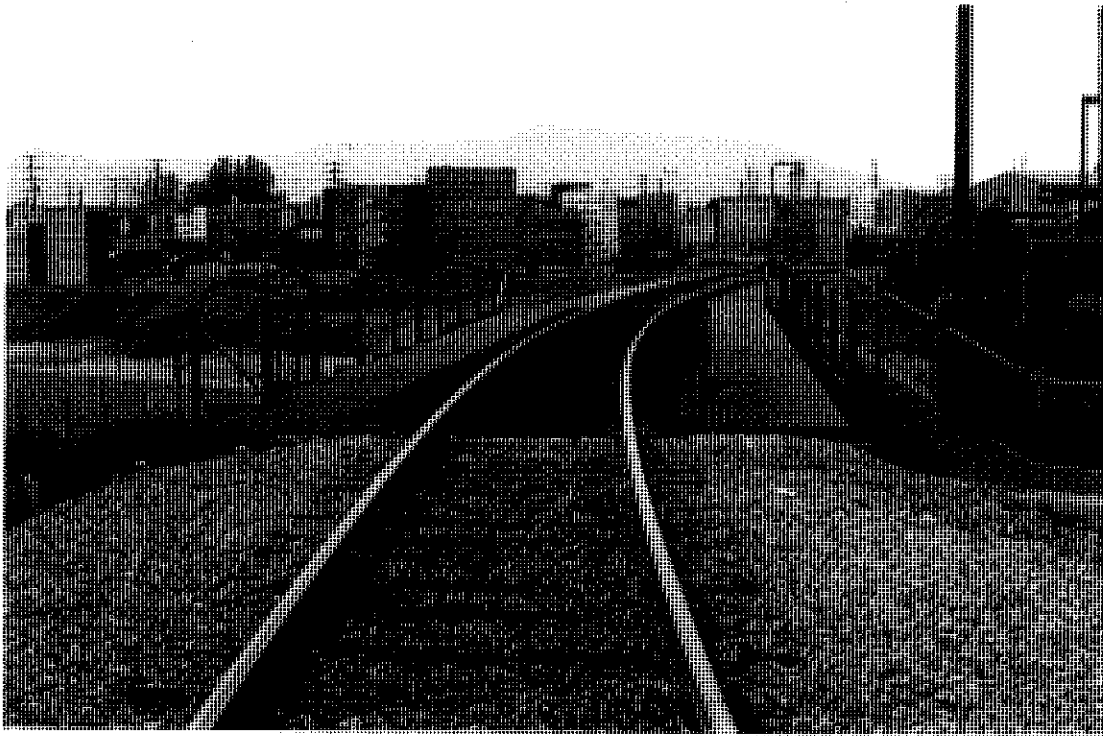
Photo 5: View of UPRR (formerly SPRR) West WYE Bridge, new wood planks line entire bridge surface, and the handrails are also brand new; view to the southwest.
