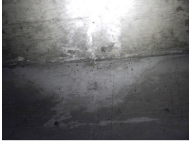
106) Los Angeles River Concrete Box Culvert West of Flower Street at Fairmont Avenue—View of extensive guano and staining along the culvert walls
