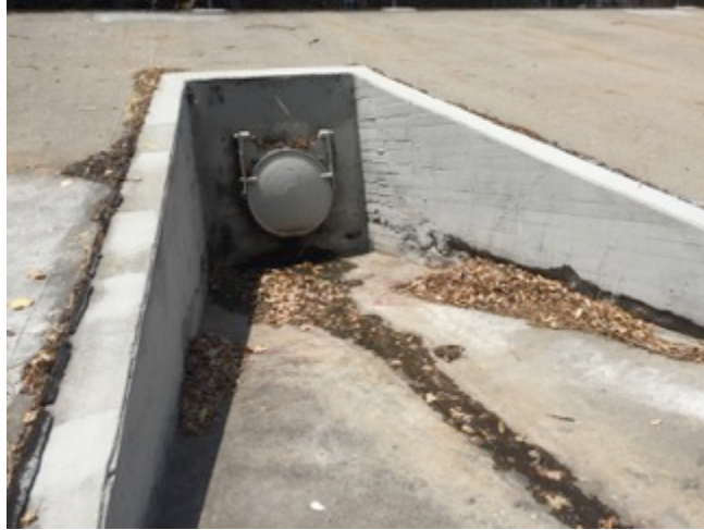
129) Los Angeles River Culverts (Various)—Representative view of concrete pipe culverts covered by steel doors present throughout the Los Angeles River
