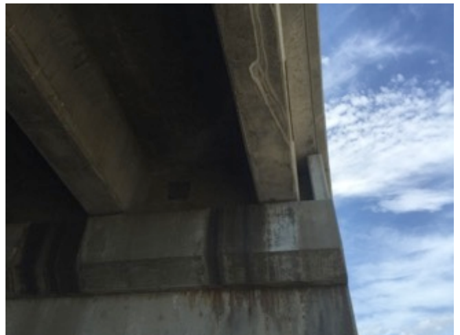
44) Western Avenue Overcrossing—View of wide crevices in the eastern abutment
