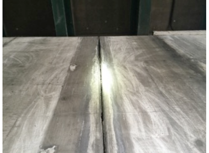
102) I-5 over Alameda Avenue—View of the vertical crevice in the concrete abutment wall where bat guano was found beneath the crevice
