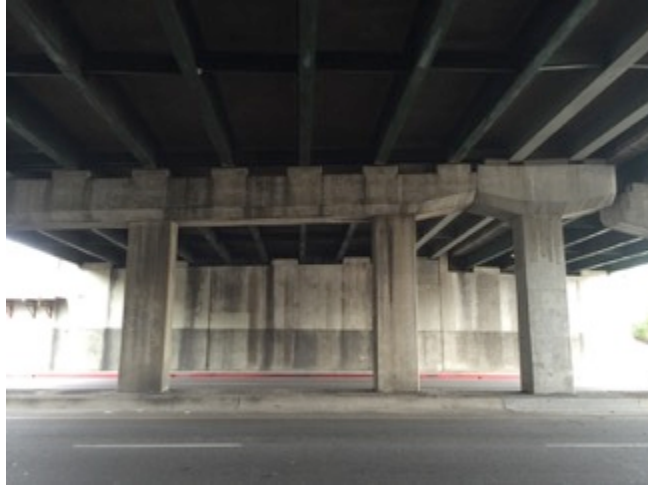
101) I-5 over Alameda Avenue—View of the bridge underside, with steel girders and vertical crevices in the concrete abutment walls
