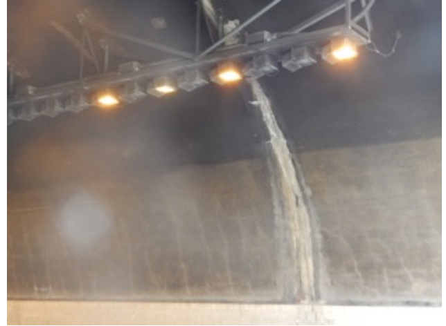
114) Figueroa Street Tunnels—View looking southwest into one of the tunnels, where a seam is visible but no crevices were observed
