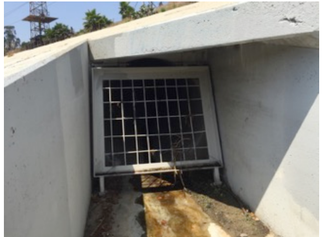
132) Los Angeles River Culvert; East Bank Southwest of Bowtie Parcel Interpretive Signs—View of the wire gate partially obstructing the entrance to the culvert
