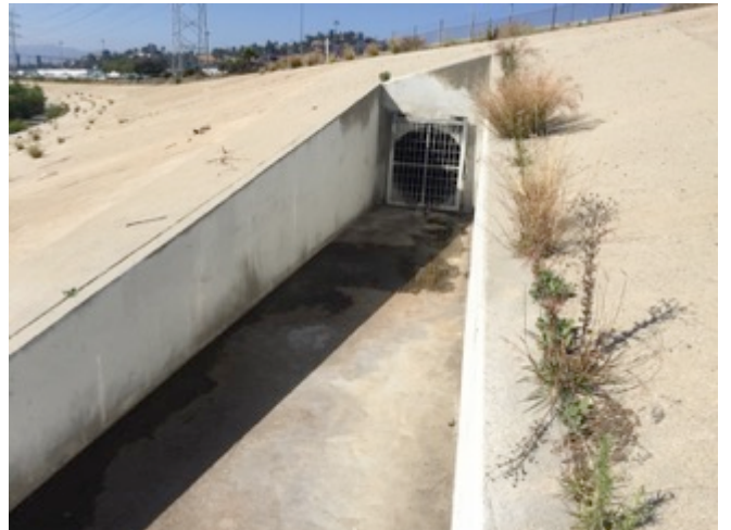
144) Los Angeles River Culvert; East Bank near Duvall Street—View of the culvert entrance with a wire metal gate
