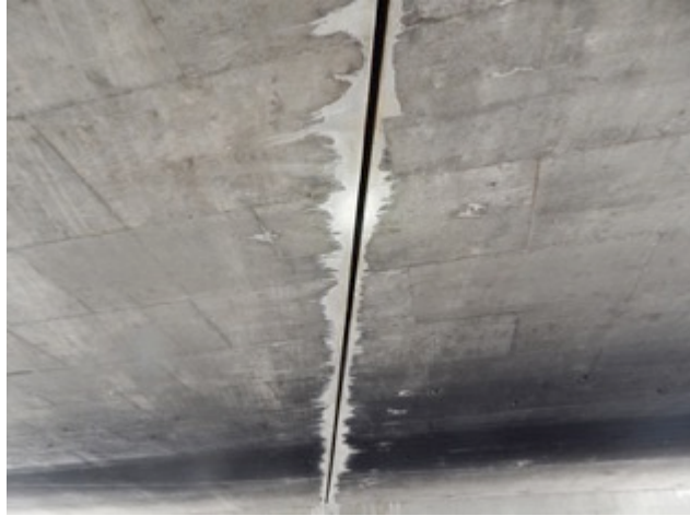
109) I-5 Colorado Street Freeway Extension over Edenhurst Avenue—View of the bridge underside with longitudinal joint opening
