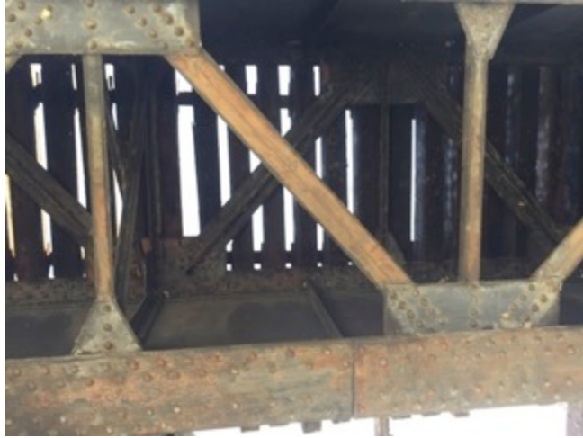
25) West Wye Southern Pacific Railroad Bridge over Burbank Western Channel—Underside of bridge with gaps between railroad ties
