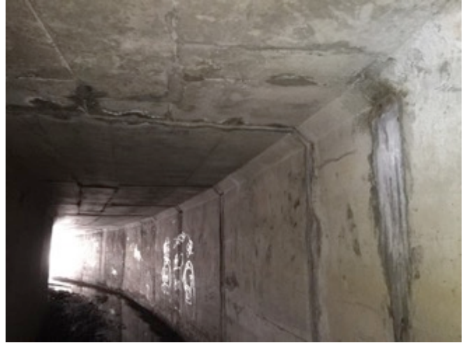
6) Double-box culvert in Burbank Western Channel near Lamer Street—Examples of extensive staining observed throughout the structure
