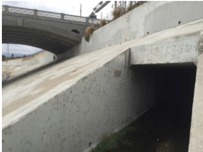
91) Main Street Bridge over the Los Angeles River— View of the concrete box culvert on the southeast side of the bridge structure
