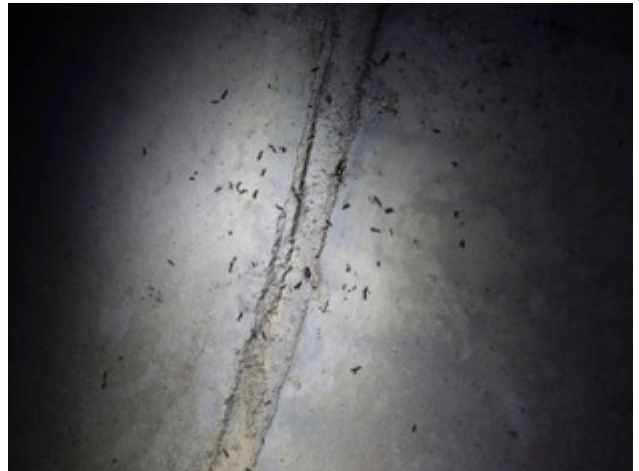
108) Los Angeles River Concrete Box Culvert East of Flower Street at Fairmont Avenue—View of one of the concentrated guano accumulations inside the structure
