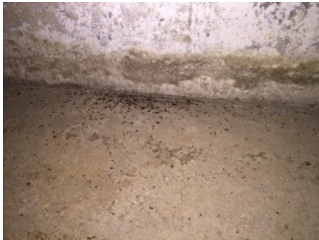
15) Elevated side culvert within I-5 culvert over Burbank Western Channel—Example of guano accumulations observed throughout the structure
