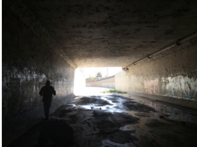
15) Elevated side culvert within I-5 culvert over Burbank Western Channel—Example of guano accumulations observed throughout the structure
