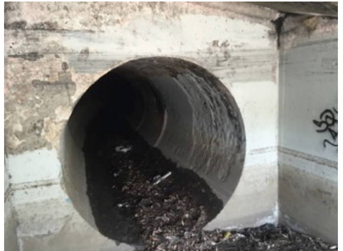
128) Los Angeles River Culvert; West Bank near Allesandro Street—View of the culvert entrance and accumulated sediment
