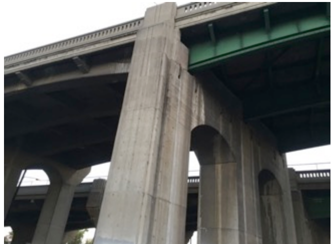
76) SR 110 Bridges—Typical view of the underside of the bridge structures with concrete and steel girders
