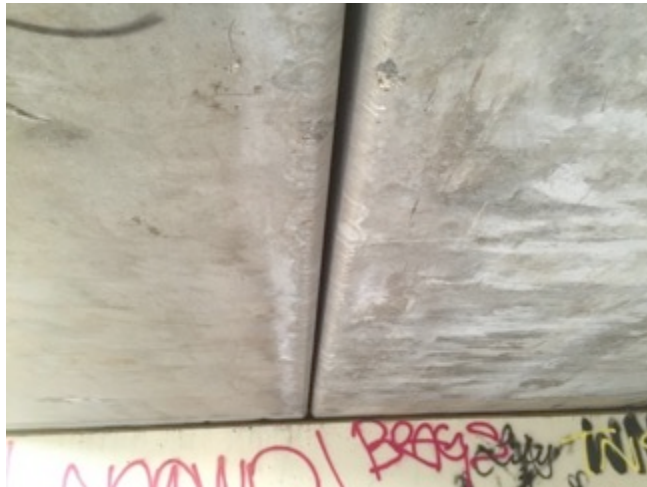
67) Metrolink Central Maintenance Facility Access Road Undercrossing—Closer view of one of the crevices in the bridge structure carrying the railroad over the Metrolink Central Maintenance Facility access road
